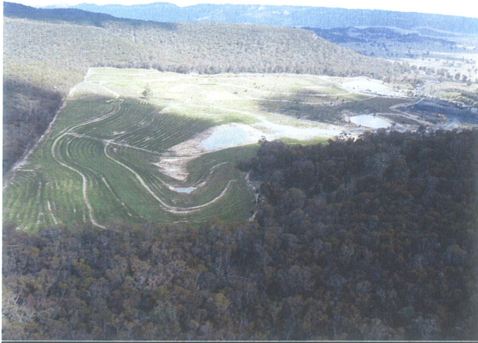
3 rd Entry Open Cut rehab
