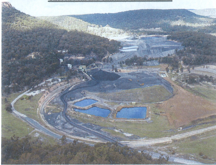
CHPP, REA and Mine Dams
