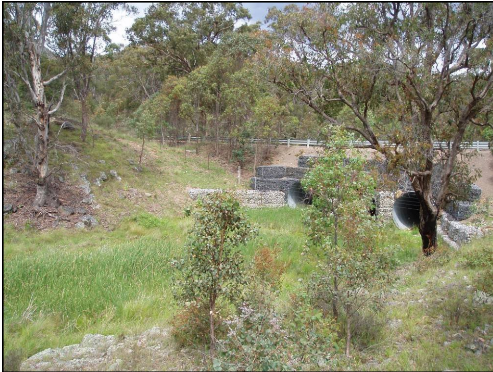
Plate 5 – Existing crossing over Airly Creek in vicinity of powerline route
