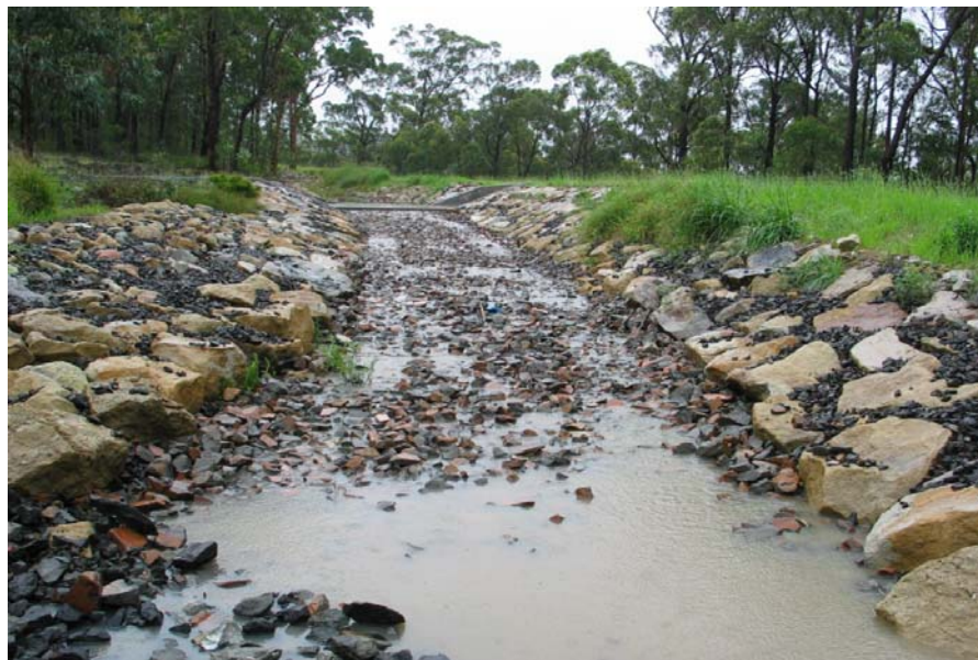
Figure 2 - Newstan SREA clean water diversion drain flow in 2011 following a heavy rainfall event.
