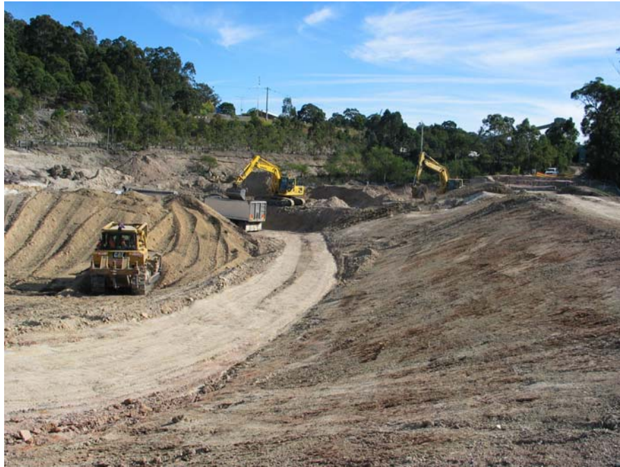
Figure 3 - Newstan FPCD construction to 50ML capacity.
