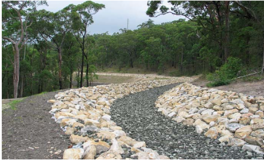
Figure 1 - A completed section of the Newstan SREA clean water diversion drain.
