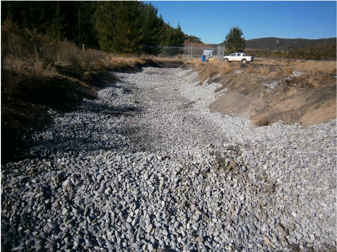
Figure 9: Ballast and Gabion Baskets installed at LDP003 coagulant dosing site
