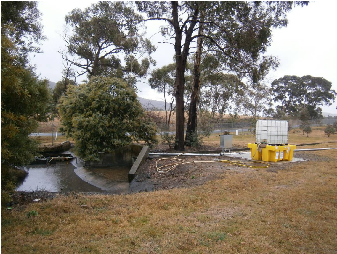
Figure 7: Automated coagulant dosing system installed at LDP002 entry point
