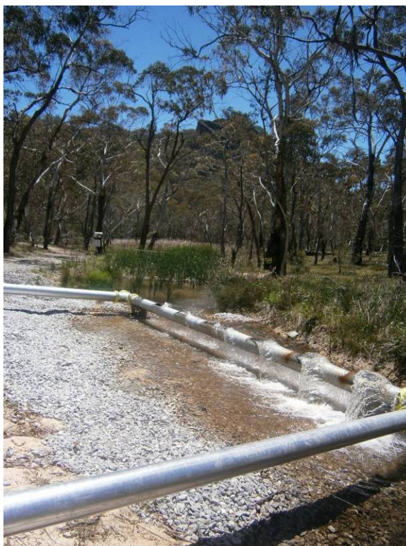
Figure 11: Galvanised pipeline installed at upstream of LDP001 to manage pH.
