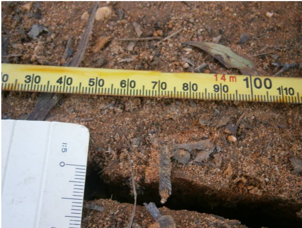
Figure 21: The maximum width of the crack measured 29/7/2011
