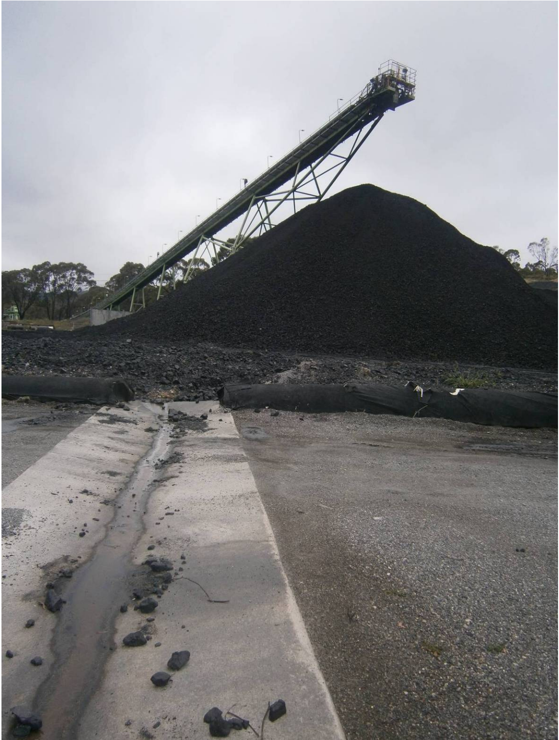
Figure 6: V Drain Installed to direct runoff from stockpile into CHP ponds
