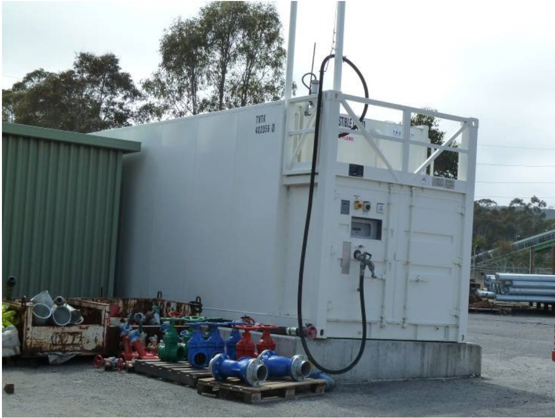
Figure 12: Self bunded Diesel tank commissioned in 2011
