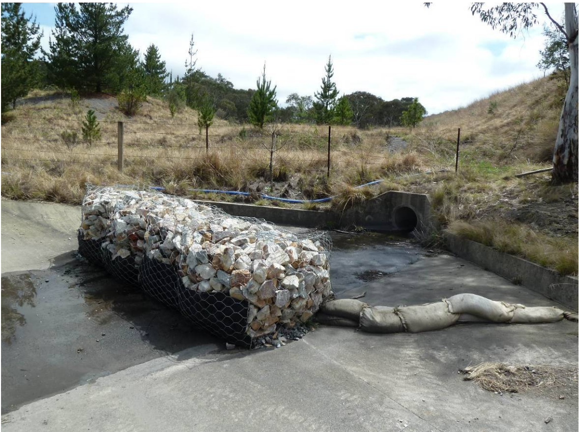
Figure 10: Geomesh lined Gabion basket installed at LDP003 primary settling pond
