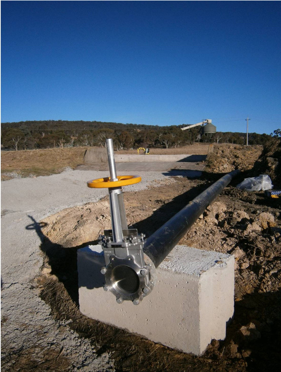
Figure 8: Controlled Discharge Valve installed at LDP002
