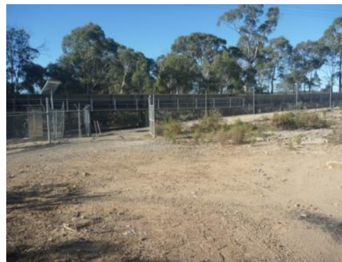
Plate 16 View south -clearing mid slope area
