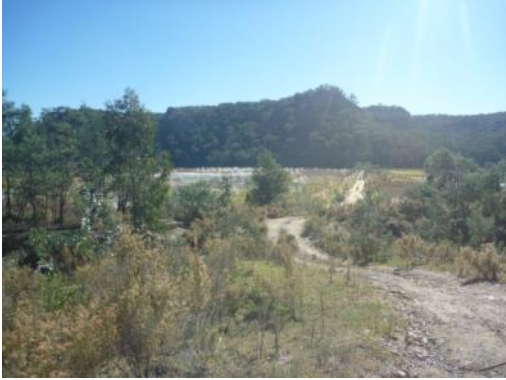
Plate 35 Modified pipeline area view north
