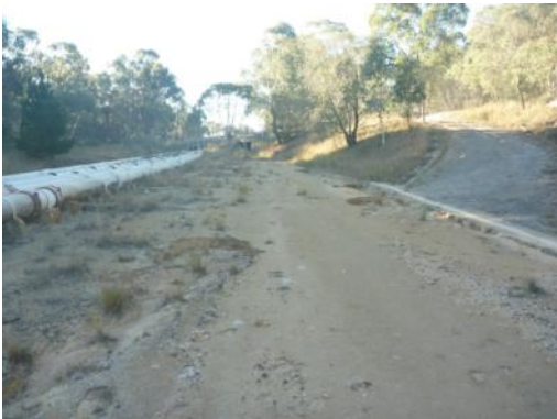
Plate 33 Existing pipeline Skelly Rd view north
