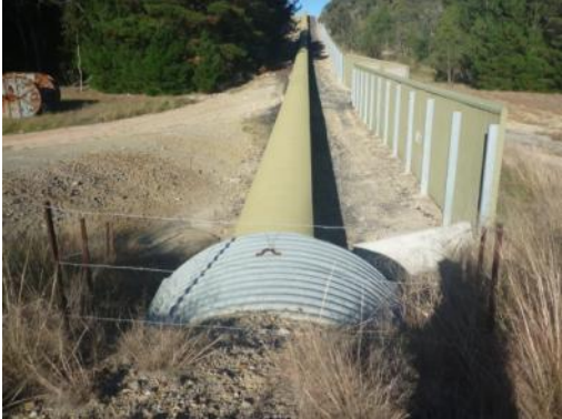
Plate 29 Conveyor area - view east
