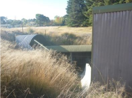
Plate 28 Conveyor Tunnel – view north
