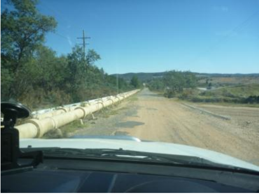
Plate 34 West of LDP009 pipeline & access road
