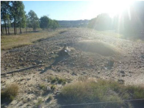
Plate 27 View west along top of conveyor tunnel
