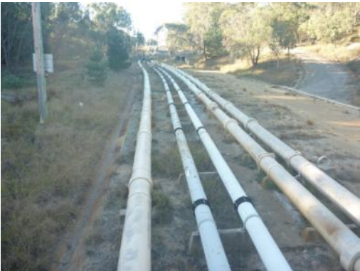
Plate 32 Existing pipeline Skelly Rd view north
