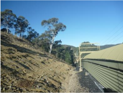
Plate 31 Conveyor near Wolgan & Skelly Roads
