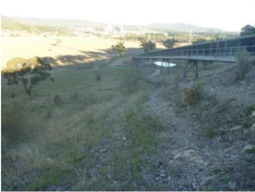
Plate 25 View north east from conveyor
