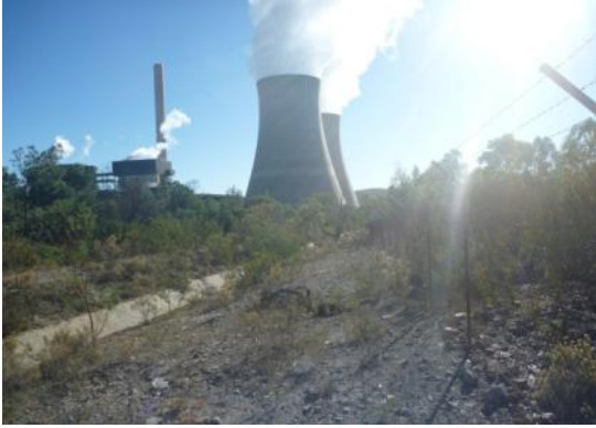
Plate 2 View north west showing culvert
