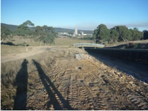
Plate 23 Overland conveyor area view east
