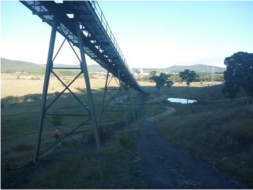
Plate 24 Modified land surface near conveyor
