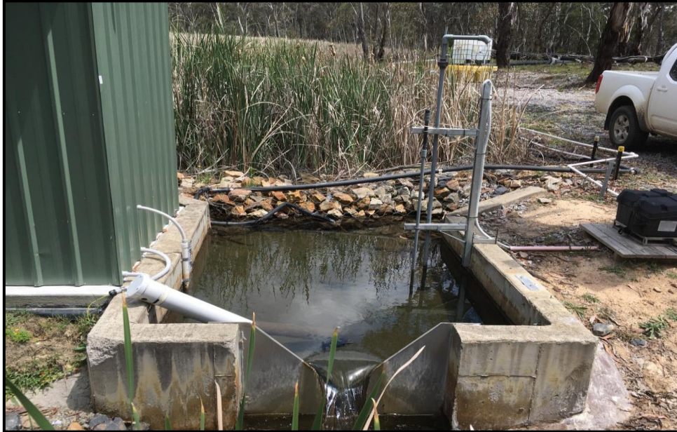
Photograph 3 – Existing V-Notch Weir at Angus Place LDP001
