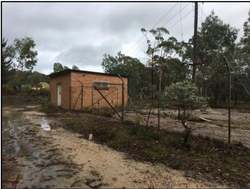
Photograph 1 – Decommissioned Switchyard Compound at Angus Place Colliery Pit Top
