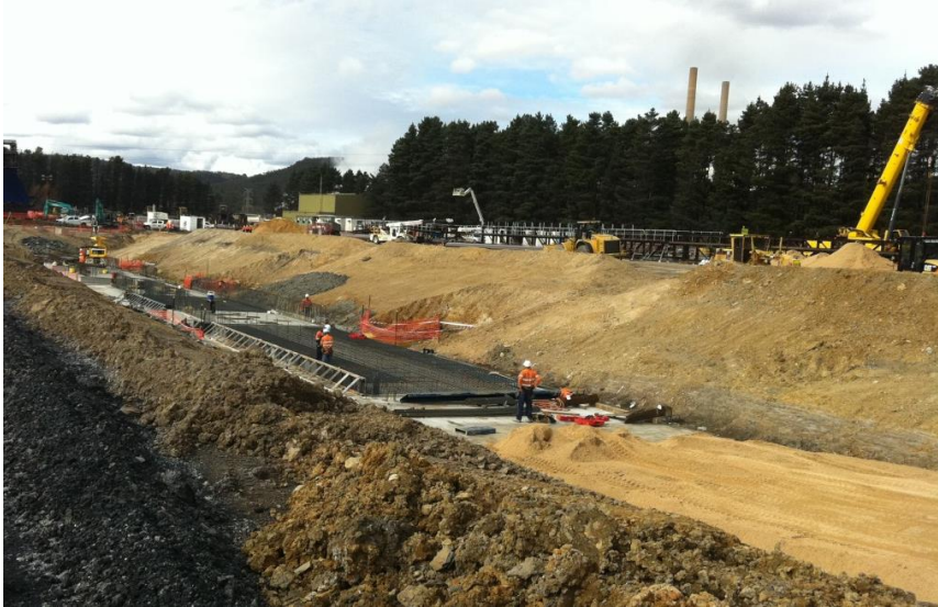
Figure 1: Construction of Reclaim Tunnel at Lidsdale Siding (August 2013)
