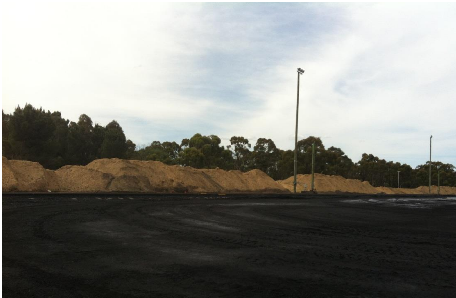
Figure 6: Bunding is to be shaped in 2014
