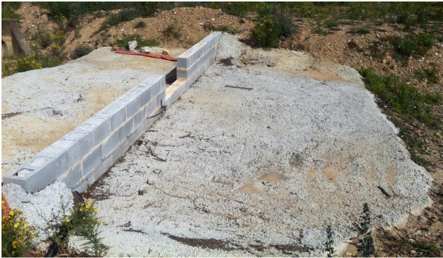
Figure 4: Licensed Discharge Point 4 at Lidsdale Siding
