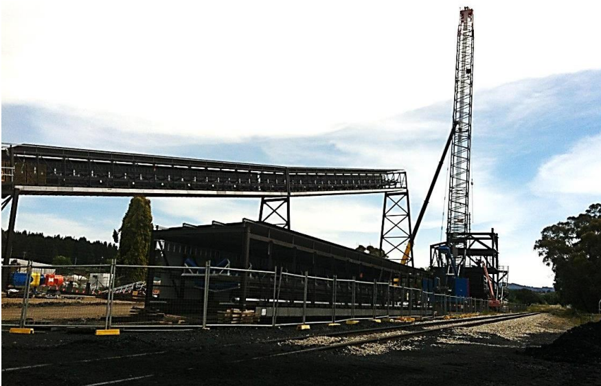
Figure 2: Construction of the Conveyor (December 2013)
