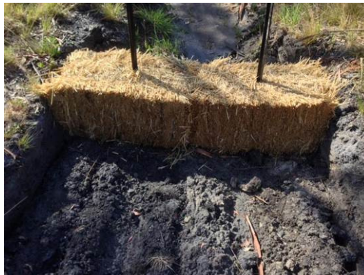
Figure 8: Hay bales in drainage lines
