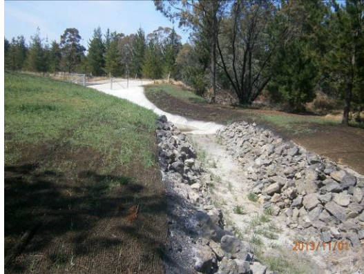
Figure 7: LDP003 new weir
