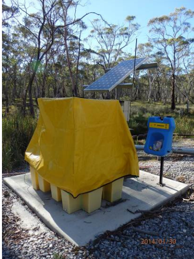
Figure 14: Eyewash station installed at LDP001
