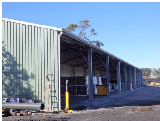
Figure 18: Mounted sprinkler at southern side of Pit Top area
