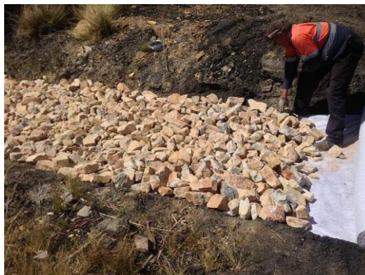
Figure 9: Drainage channels lined with terra-ferma and gabion rock
