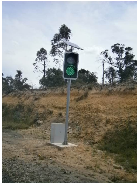
Figure 31: Traffic Management system installed on Wallerawang Haul Road
