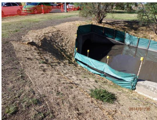
Figure 6: Carpark Culvert improvement area
