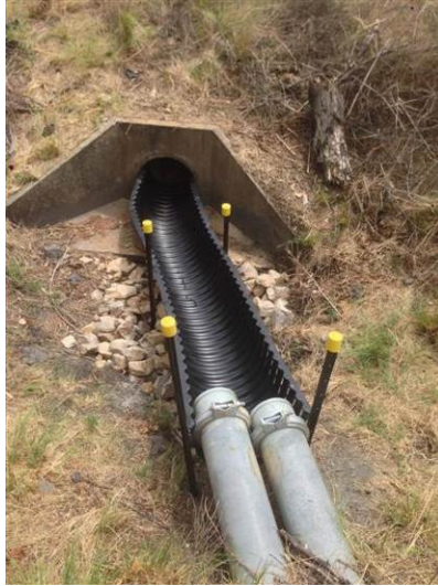
Figure 10: Direct water delivery into pipes
