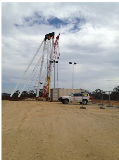
Figure 3: Ventilation Shaft Drilling area
