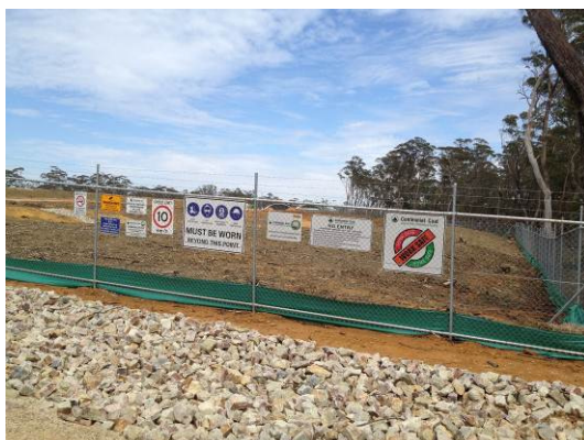
Figure 2: Entrance into the Ventilation Facility site
