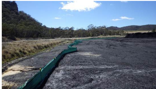
Figure 11: Installation of sediment fence around stockpile area
