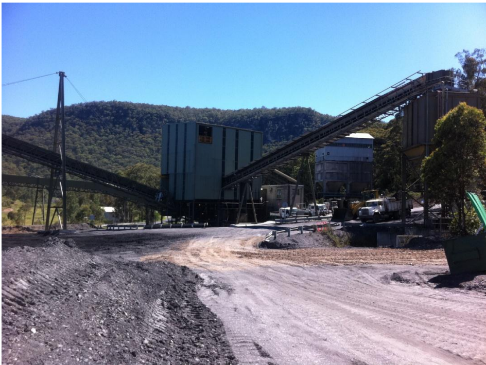
Figure E4 Shielded Conveyors at CHPP
