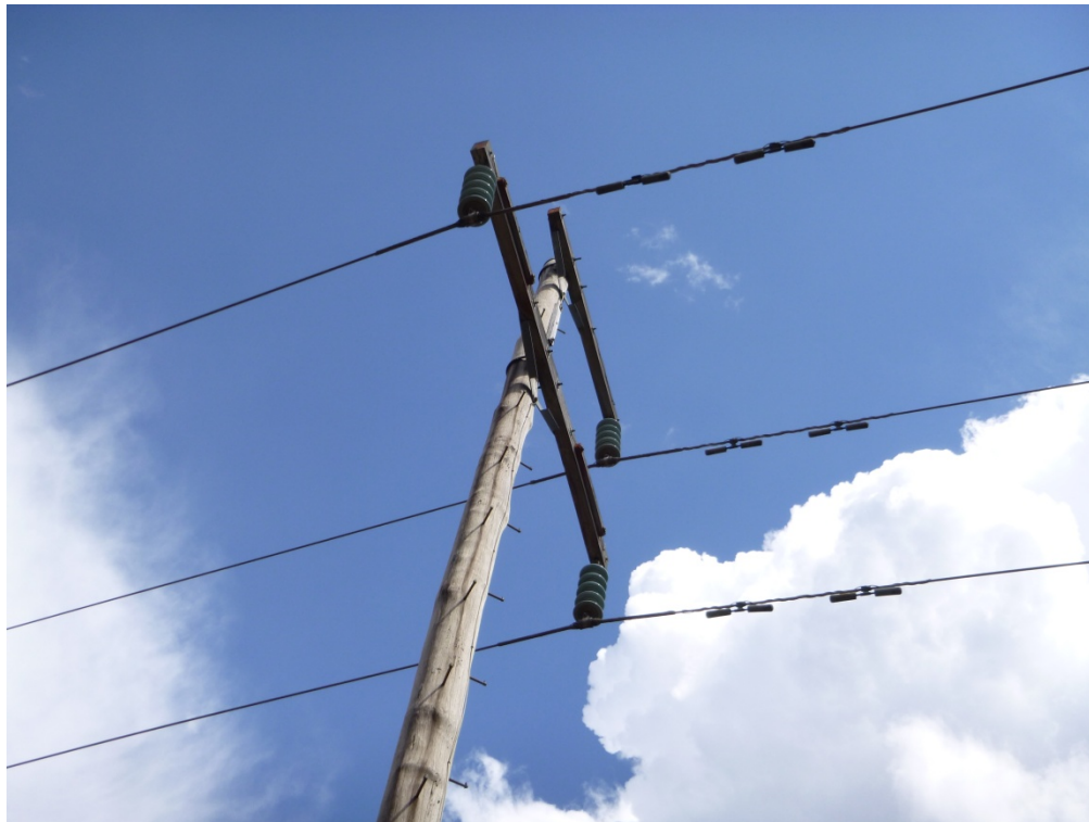
Figure 3 - Structure 207 pole top
