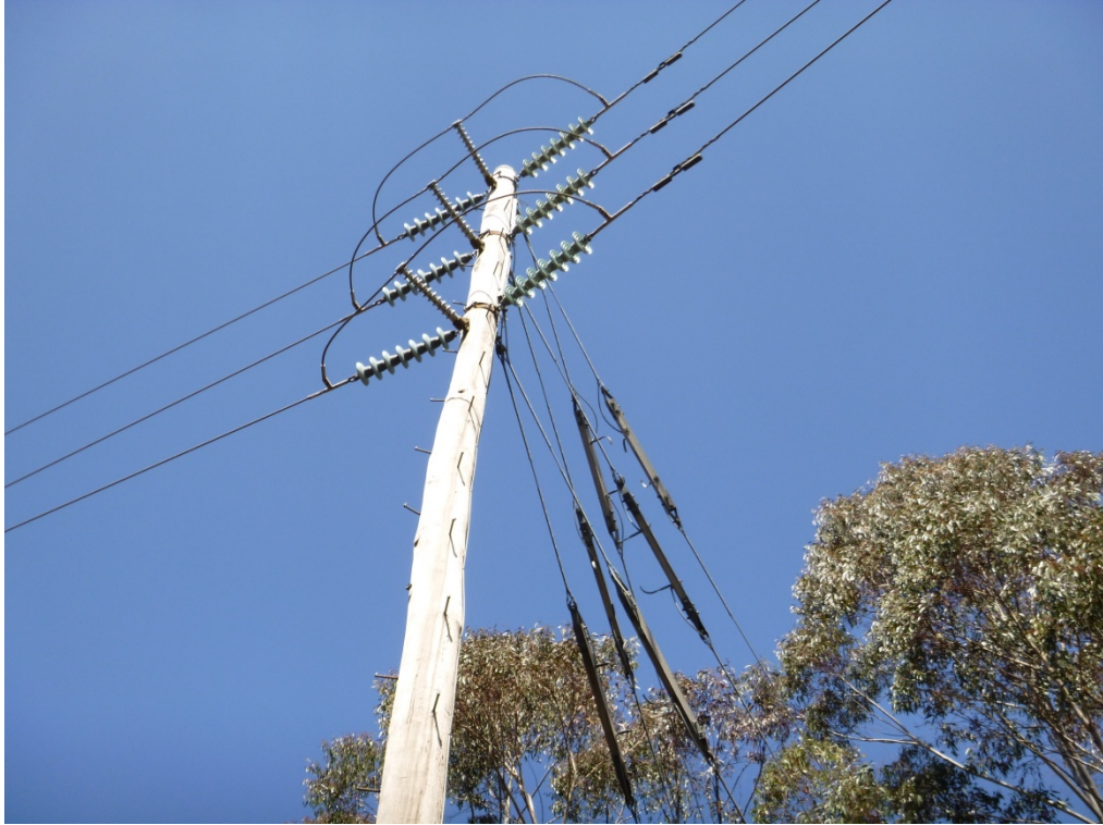
Figure 2 - Structure 206 pole top
