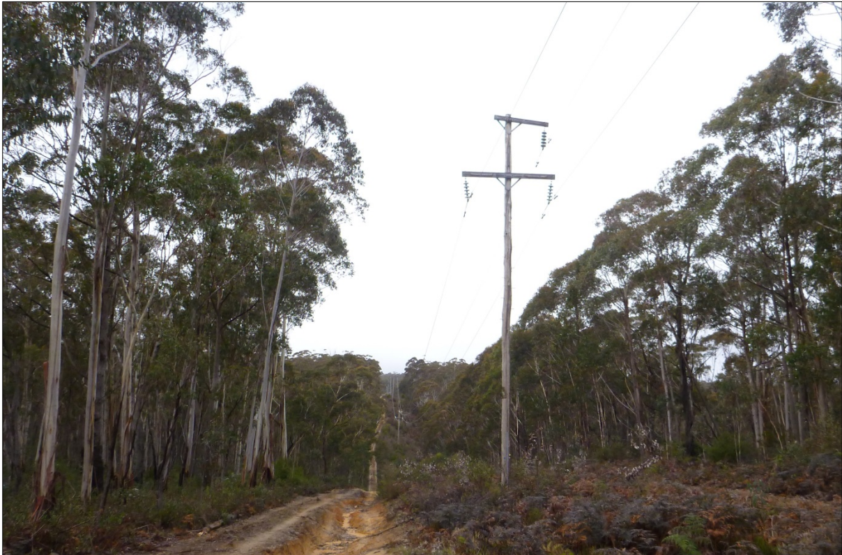
Plate 1. Endeavour Energy 66kV Powerline at Angus Place
