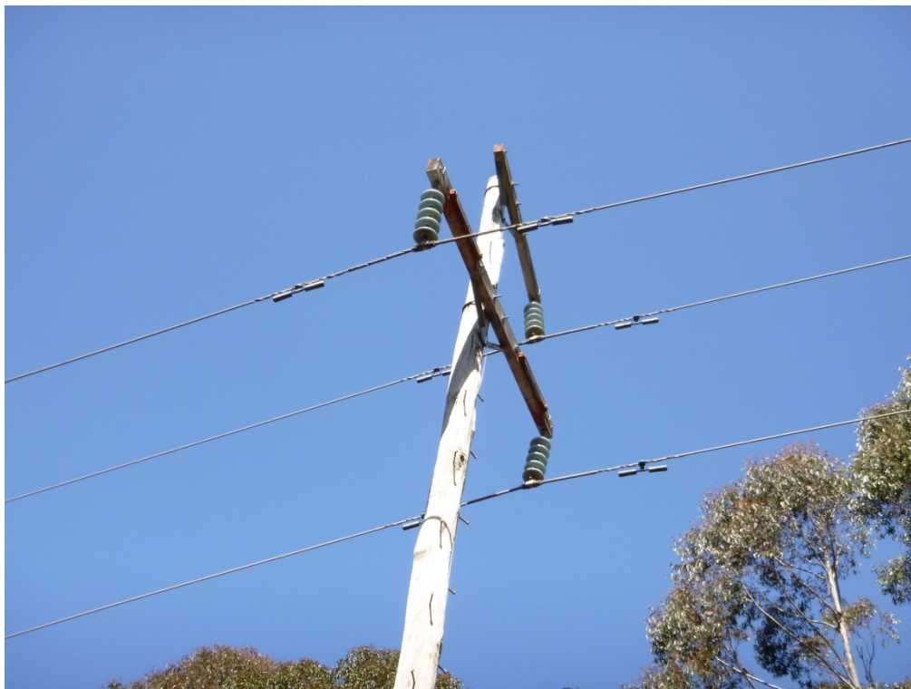
Figure 1 - Structure 205 pole top
