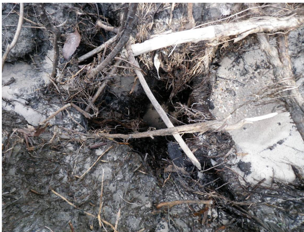
Figure 1.58 Cavity Site - No Mine Water Discharge on 1 May 2009 – Hole Where Water Loss Occurred
