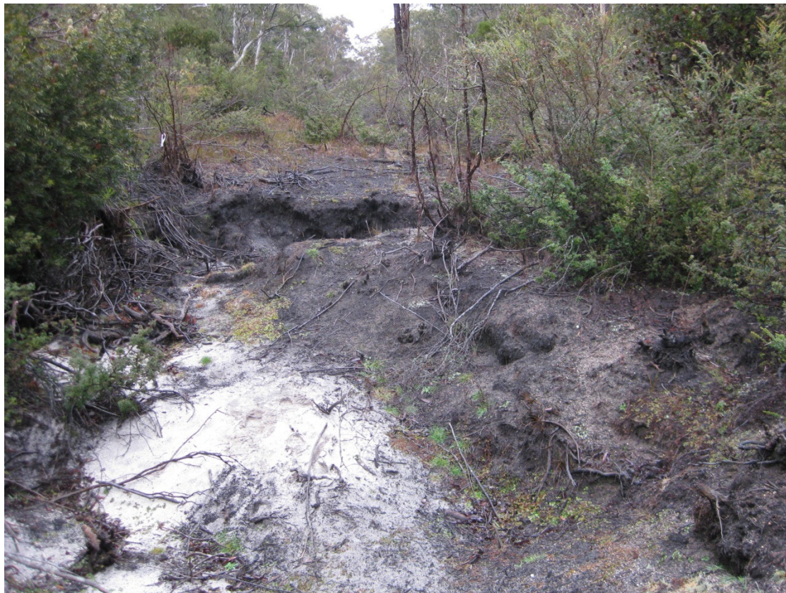
Figure 1.17 – Location 7-9 Northern Slumping Site on 28 June 2013 – note vegetation impacts
