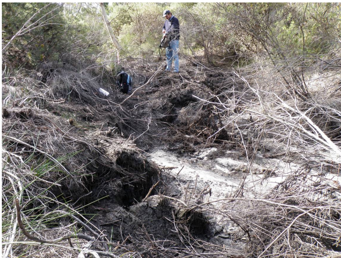
Figure 1.16 - Location 7-9 Northern Slumping Site - No Mine Water Discharge on 1 May 2009
