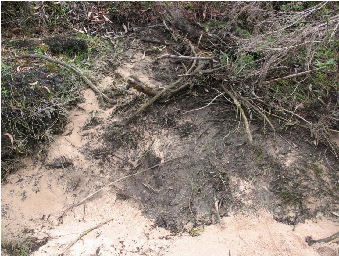
Figure 8.18 Northern Slump Site 16 June 2008 – Between Major Emergency Discharges
