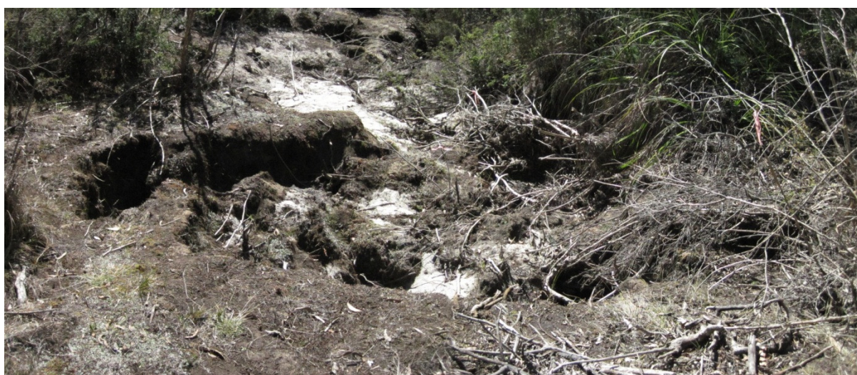
Figure 8.31 EWS Northern Slump - 12 September 2012
