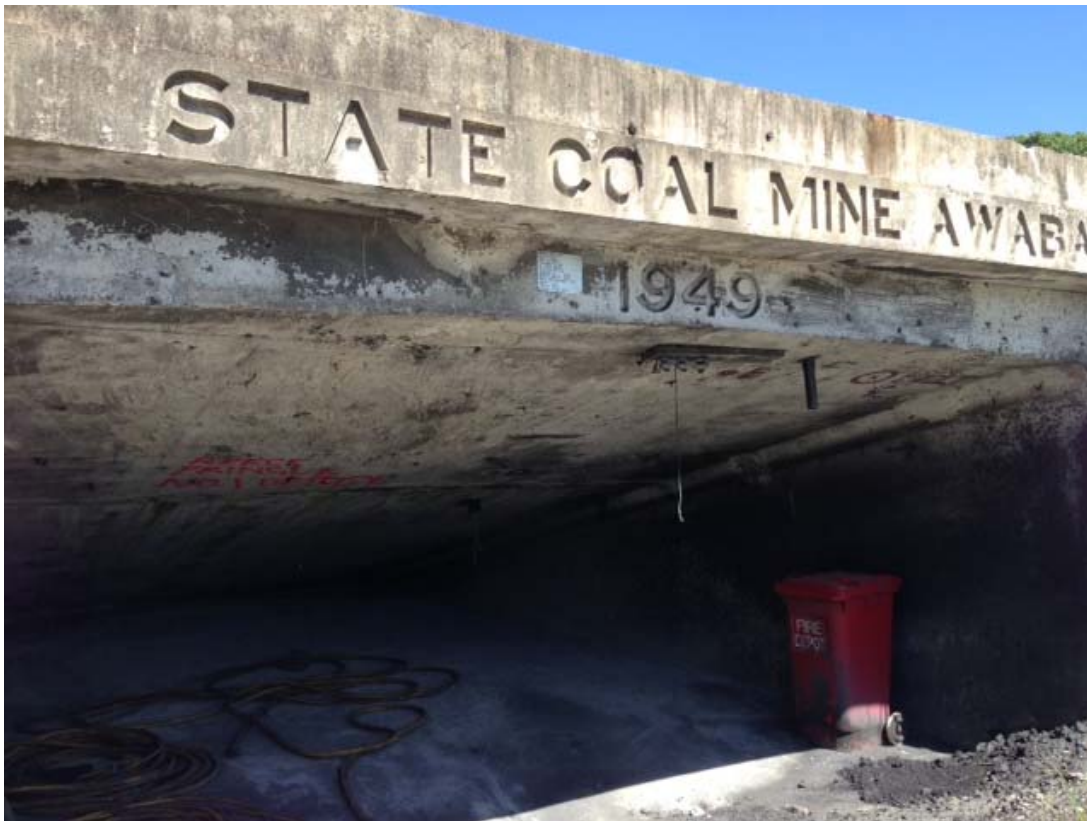
Figure 5: Sealed Mine Entry
