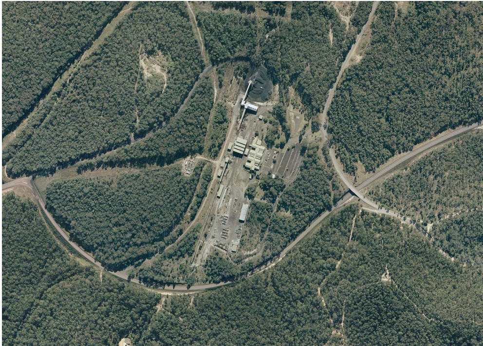
Figure 1: Aerial photograph of Awaba Colliery Surface Facilities
