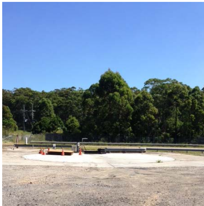
Figure 6: Decommissioned bin & sealed shaft
