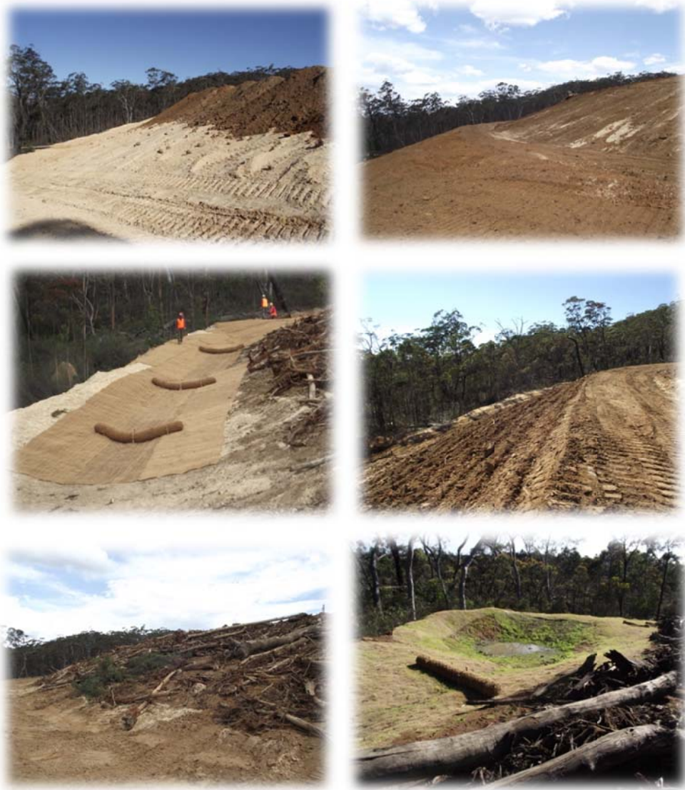
Figure 88 Rehabilitation Progress of REA IV in 2012
