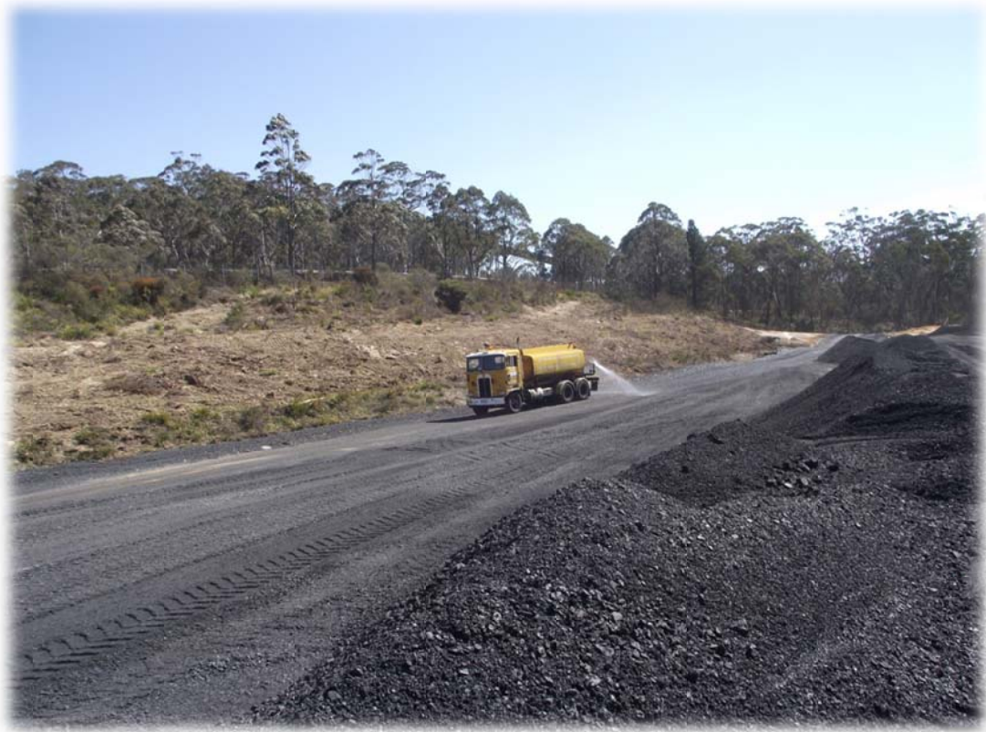
Figure 11 Water Cart in use at Clarence Colliery REA IV
