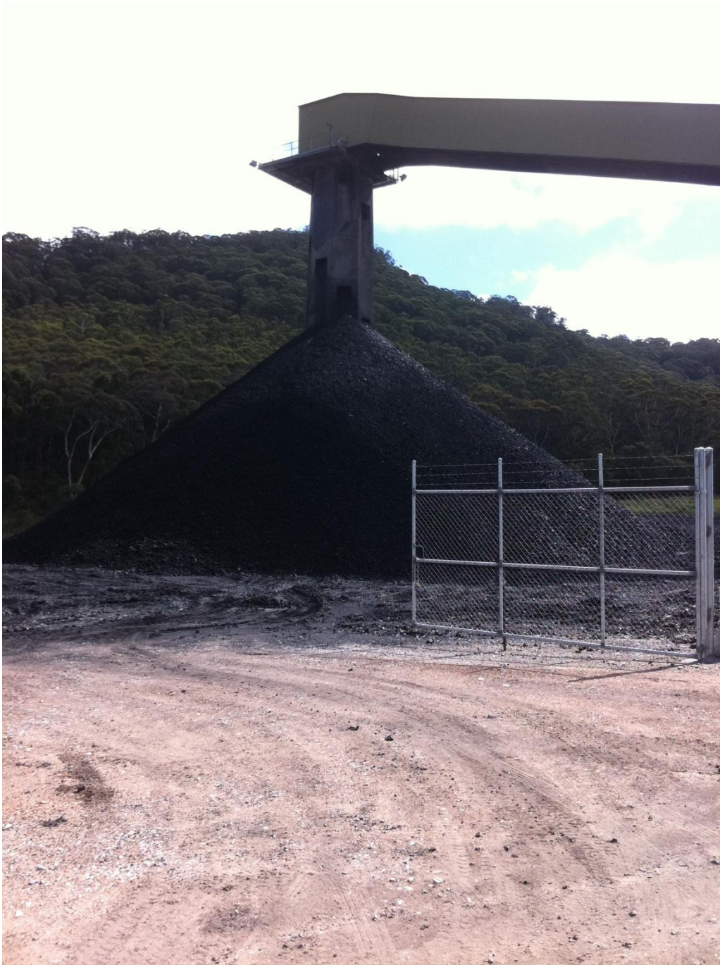
Figure C2 Water Spray on ROM Stockpile Load Point
