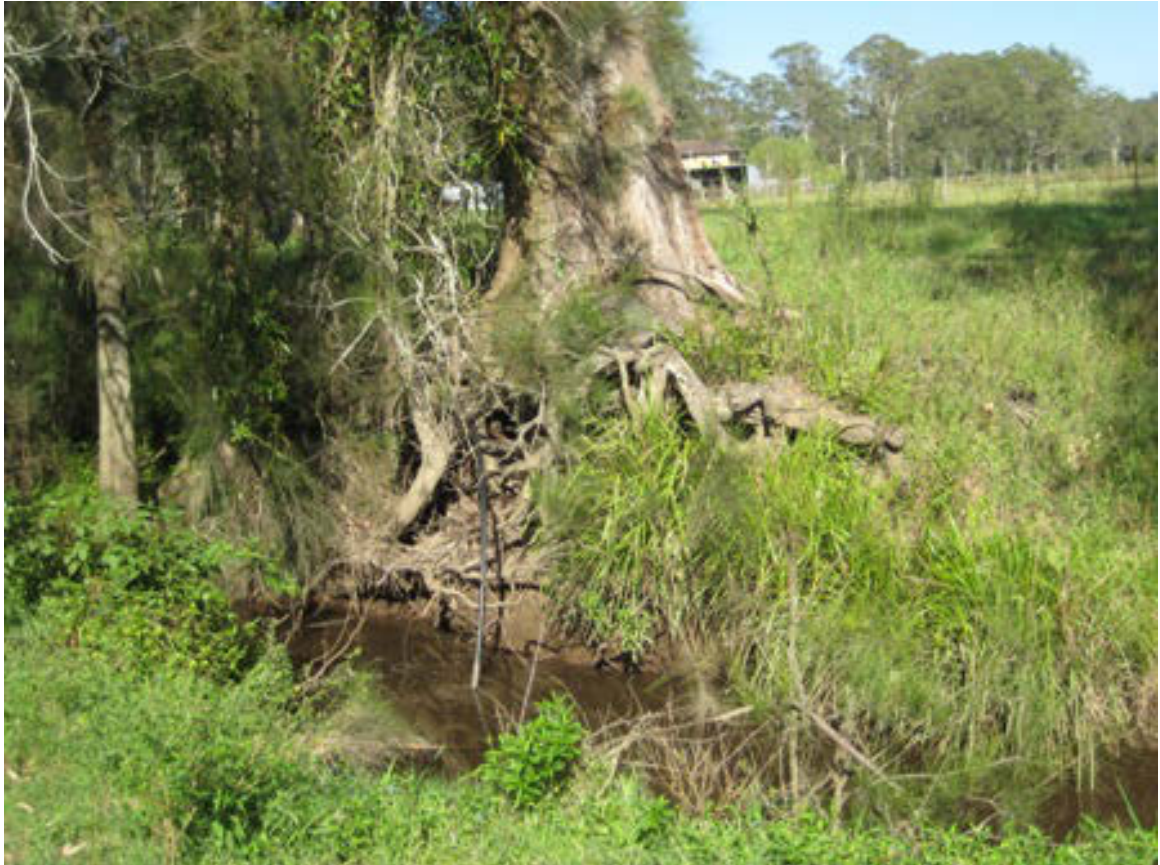
PT12 – Flank St Creek December 2008
