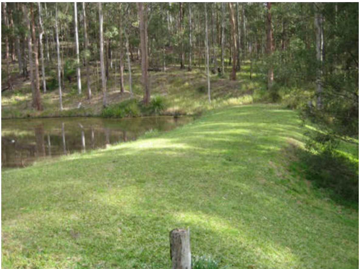
PT21 MG3 1HD Dam Wall Property Ref 108 –June 2008
