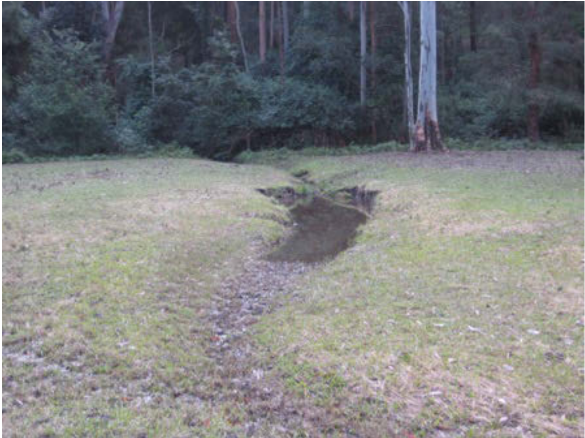
PT26 MG4 1HD Drainage line property ref 109 June 2008
