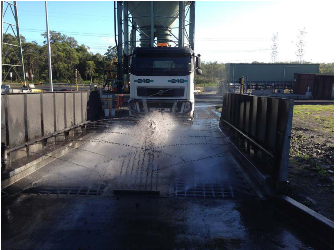
Plate Six: Cooranbong Truck Wheel Wash installed in October 2013.
