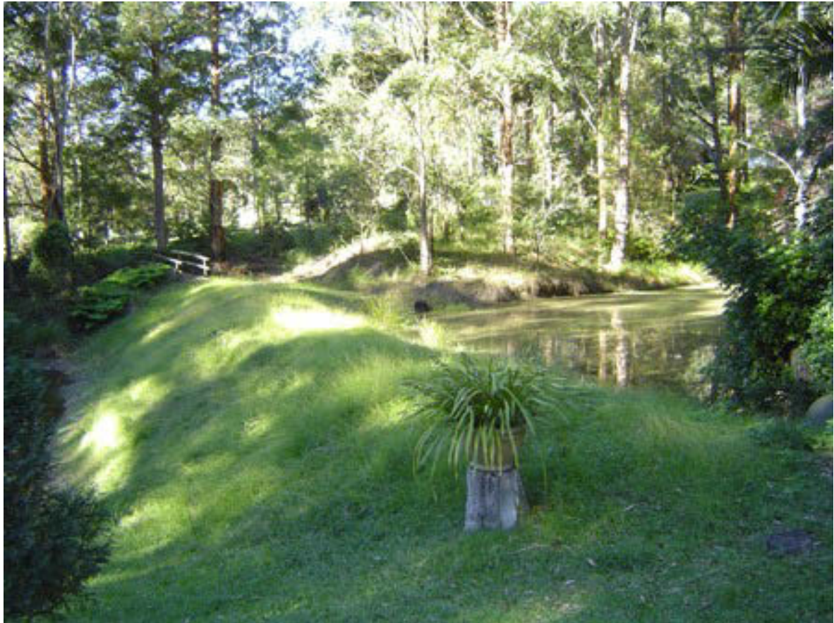
PT23 Dam Property Reference No. 109 April 2007
