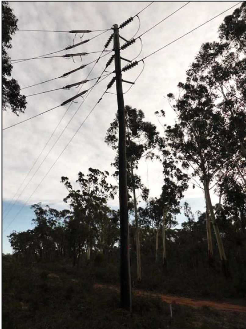
Figure 6. Power Pole #206 Facing North – 9 June 2015
