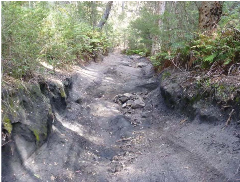
Plate 15 Section of access track to ARP13 / ARP13SP, ARP14, ARP15 / ARP 15SP, ARP15A and the V-notch weir requiring regrading
