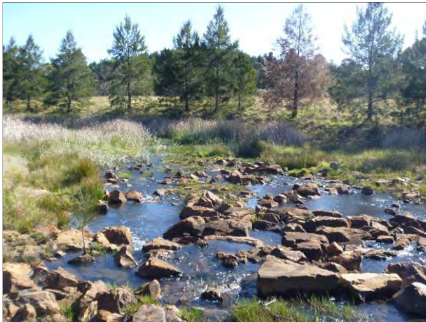
Plate 12 Creek bed stabilisation at Coxs River, Commonwealth Colliery.
