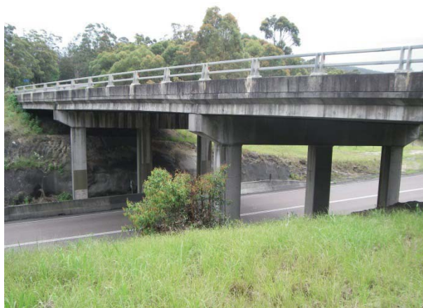
Plate 5 - Bridge WR-BR2 where the Wilton Road crosses the Haul Road
