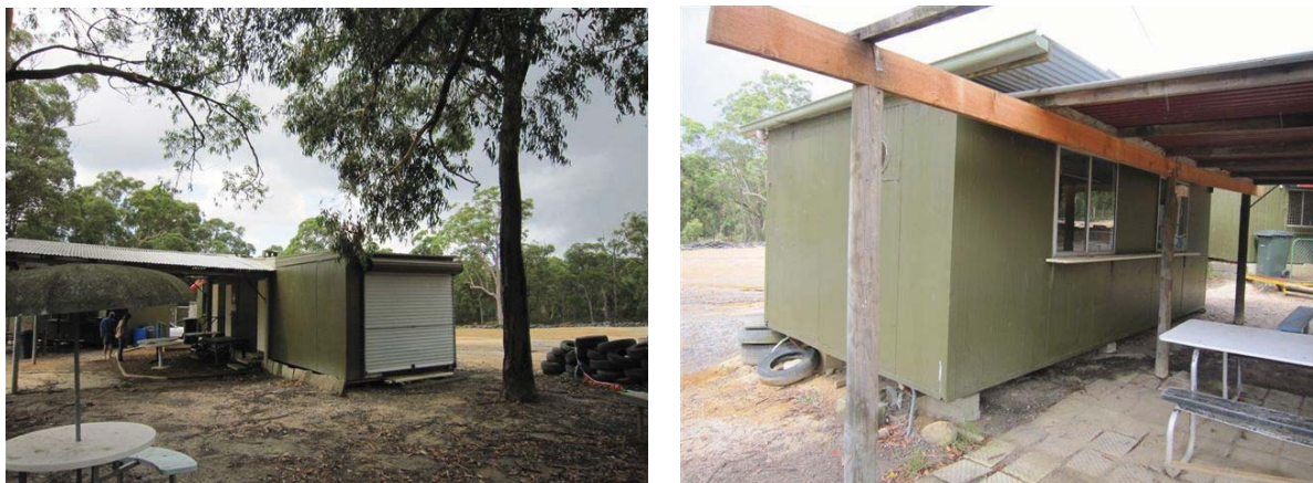
Plate 17 - Building Structures at Westlakes Automobile Club (Courtesy of Northrop Engineers)
