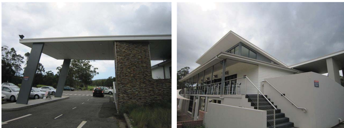
Plate 13 - Photographs of the Main Club House (Refs. TR001_pa01 and TR001_pa02) (Courtesy of Northrop Engineers)
