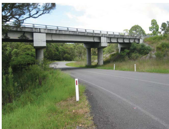
Plate 6 - Bridge CR-BR2 along Cessnock Road (Courtesy of ACOR Appleyard)
