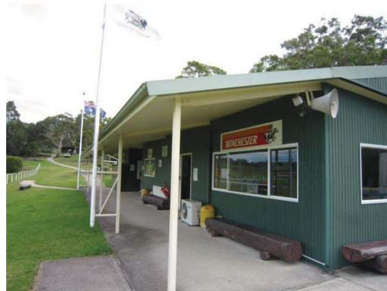
Plate 14 - Main Club House (Ref. AW001_pa01) (Courtesy of Northrop Engineers)
