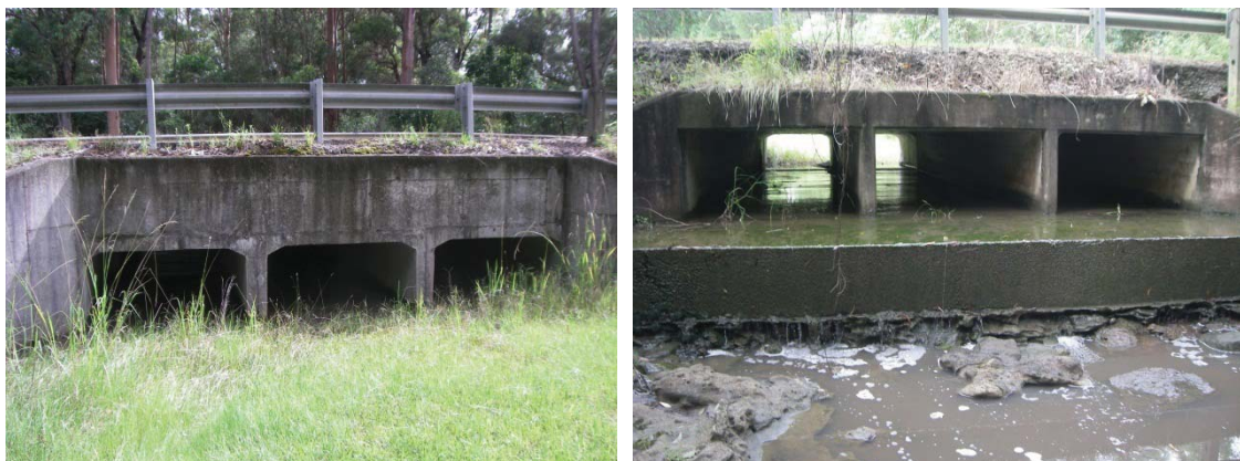
Plate 7 - Photographs of Box Culvert WI-C3 along Wilton Road
