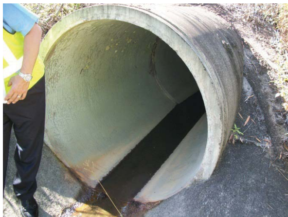
Plate 8 - Photograph of Culvert HR-C1 along the Mine Haul Road (Courtesy of ACOR Appleyard)
