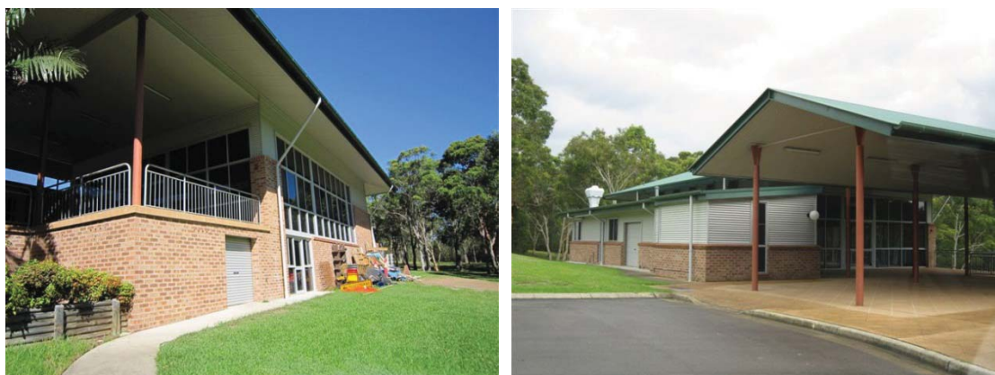
Plate 12 - Photographs of the Main Hall (Ref. TR003_pa01) (Courtesy of Northrop Engineers)
