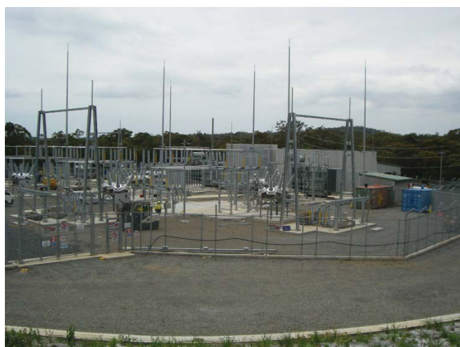
Plate 9 - Photograph of the 132/11 kV Substation
