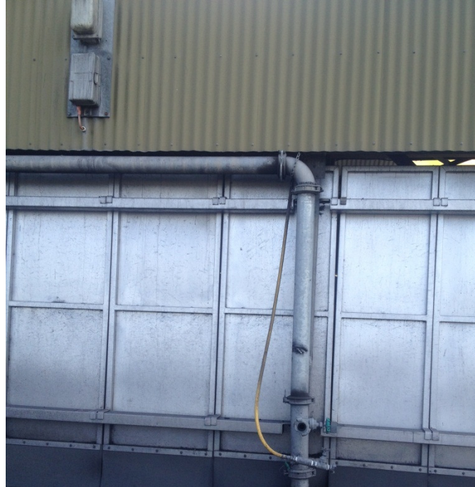
Figure 10: Noise cladding installed in 2014
