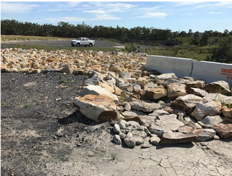
Photo 3.7 Additional rip rap at the top of the downstream batter
