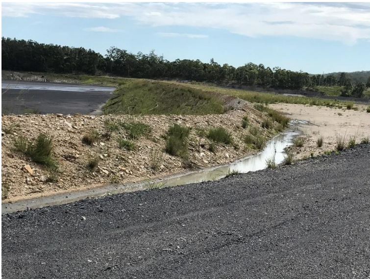
Photo 3.4 Pooled water at the base of the upstream batter windrow
