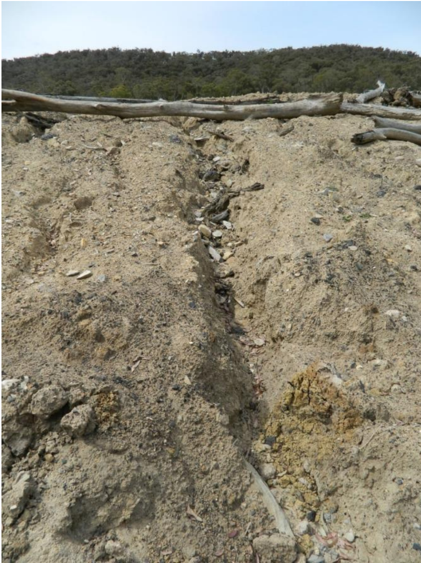
Photo 19: Minor erosion present at the end of Stream 3 sediment control structure
