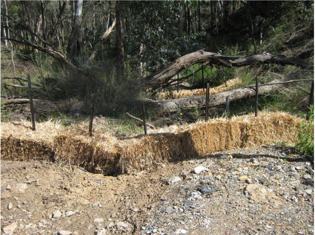
Photo 24: Hay bales were recently installed
