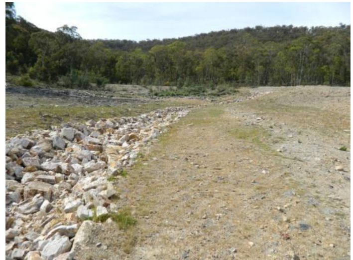
Photo 12: Examples of a well designed and well implemented erosion and sediment control structure in place at Stream 3
