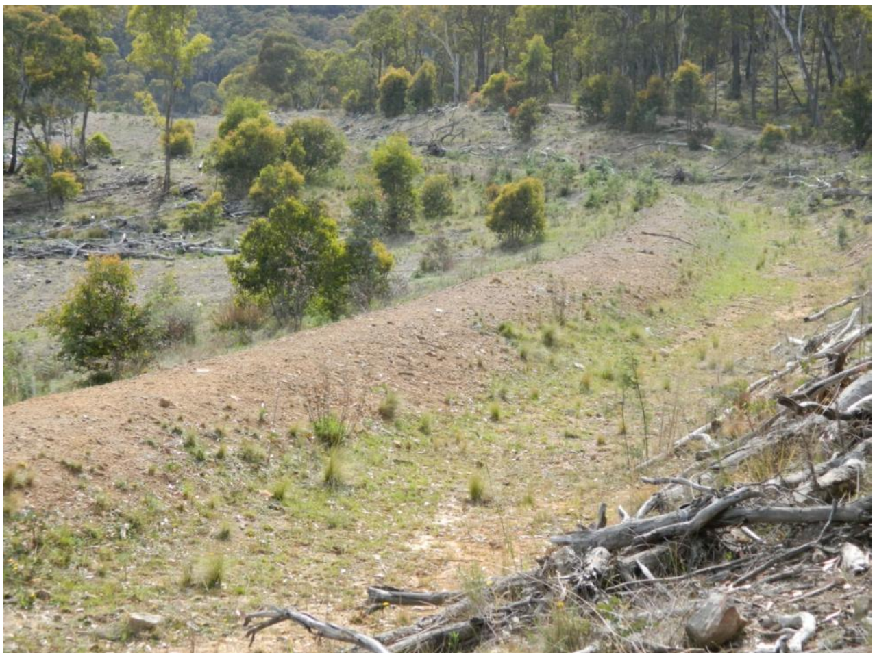
Photo 2: A successful clean water system showing no signs of erosion
