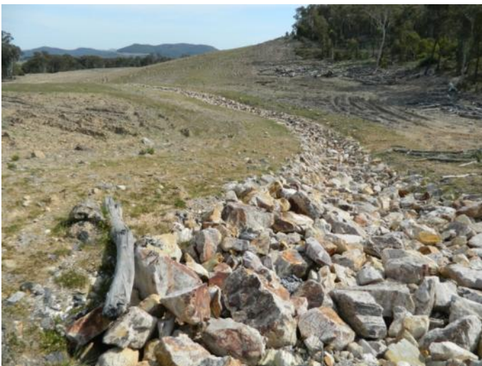
Photo 12: Examples of a well designed and well implemented erosion and sediment control structure in place at Stream 3
