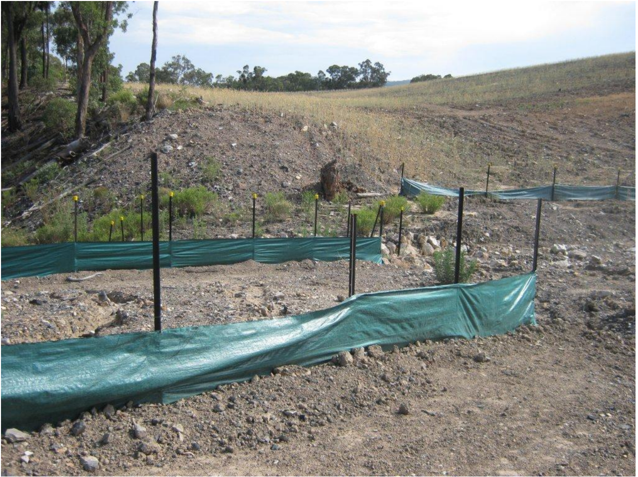
Photo 23: Erosion and sediment fencing was recently installed
