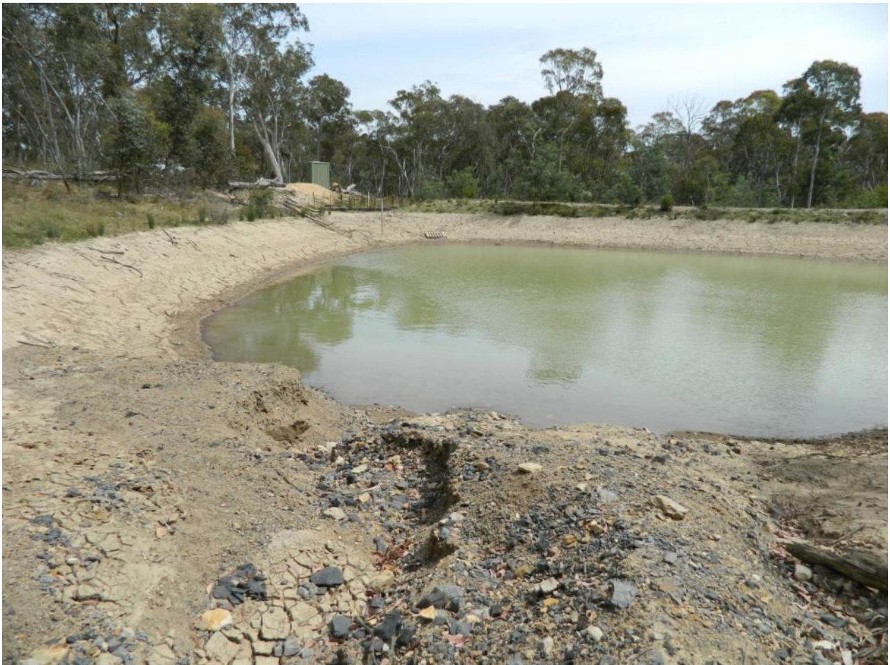
Photo 18: Sediment Dam 1 showing signs of minor erosion
