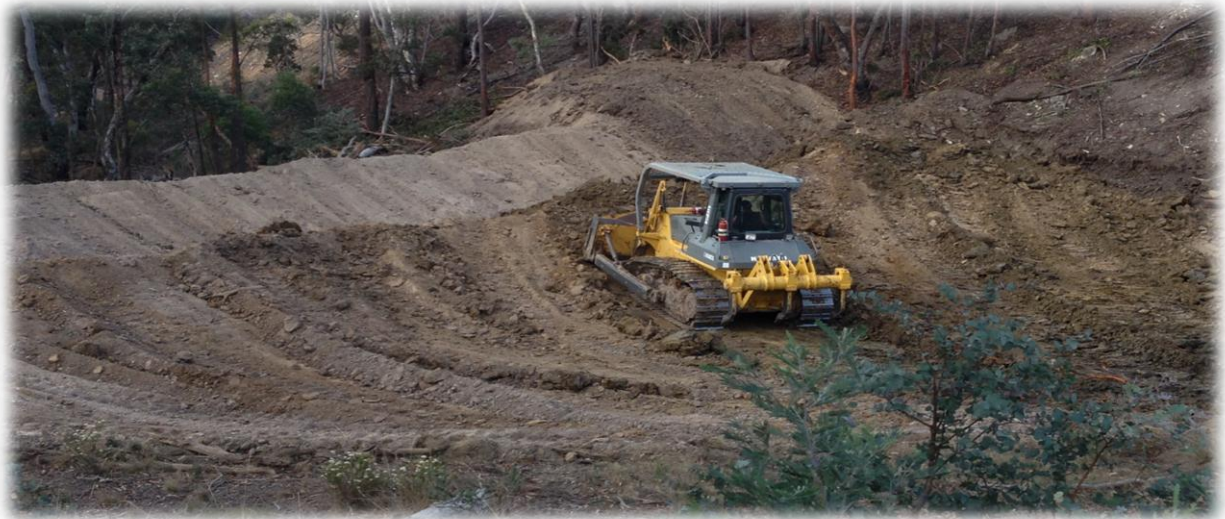
Figure 2. Preliminary Sediment Dam 1B: resizing work during the reporting Period
