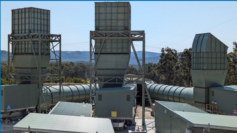
Ventilation fans and attached silencers 1 and 2 at Mandalong South Surface Site
