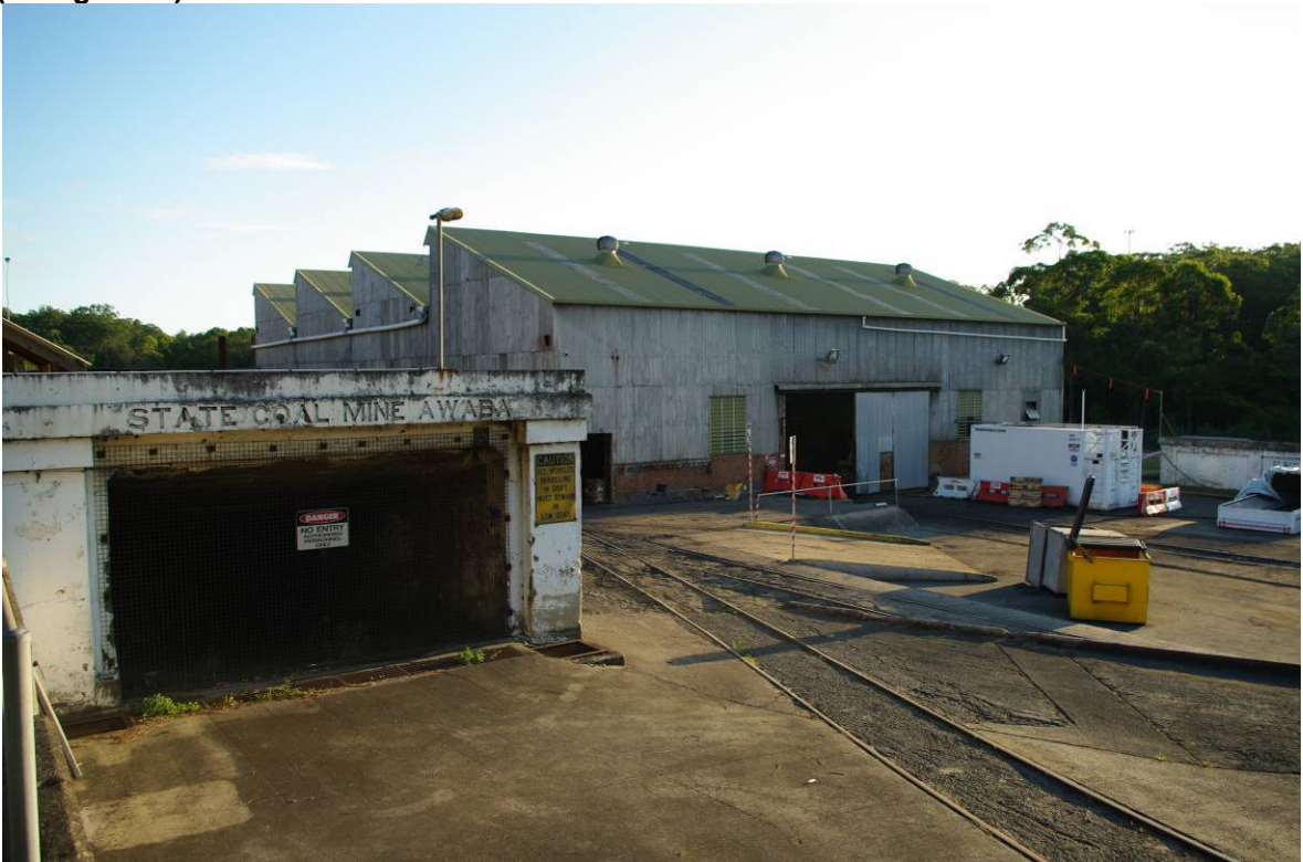
Plate 6-3 Drift portal with State Coal Mine Awaba inscription (foreground), station workshops (background).
