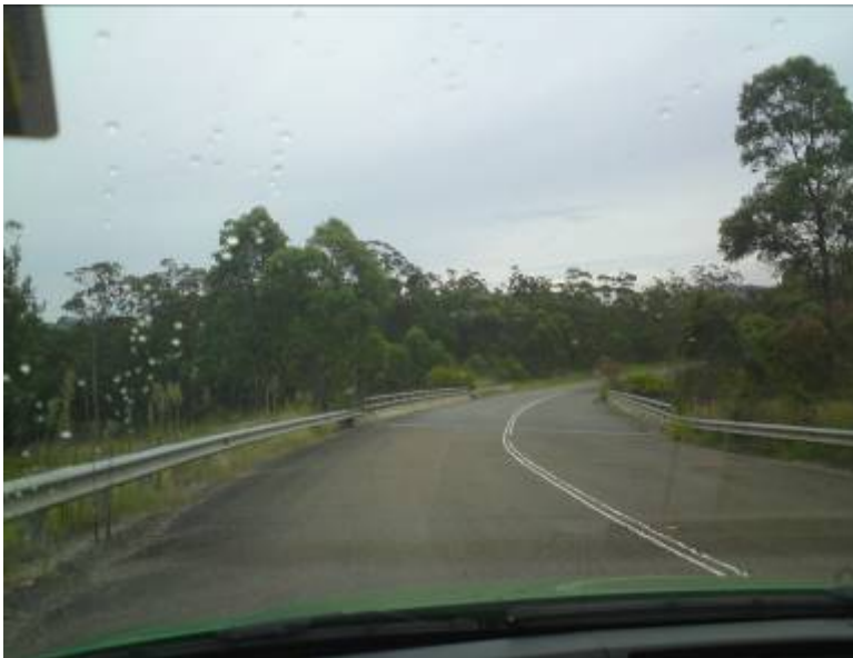
Figure 4-1 Wilton Road at the haul road overbridge, looking north
