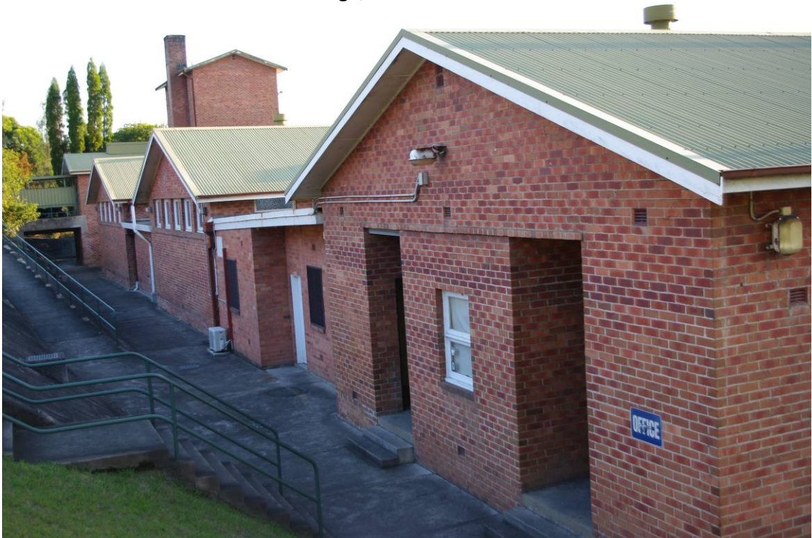
Plate 6-2 Awaba administration buildings, built c1950
