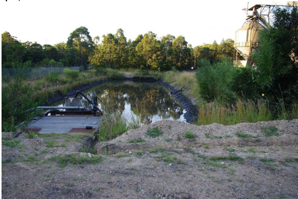
Plate 6-1 Pollution Control Dam (PCD), as inspected by RPS, ADTOAC and WNAC on 16 th of April, 2010
