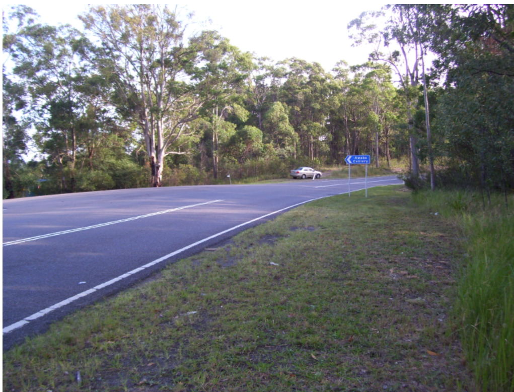
Figure 6-1 Eastern verge showing substandard shoulder and tree in 'clear zone'
