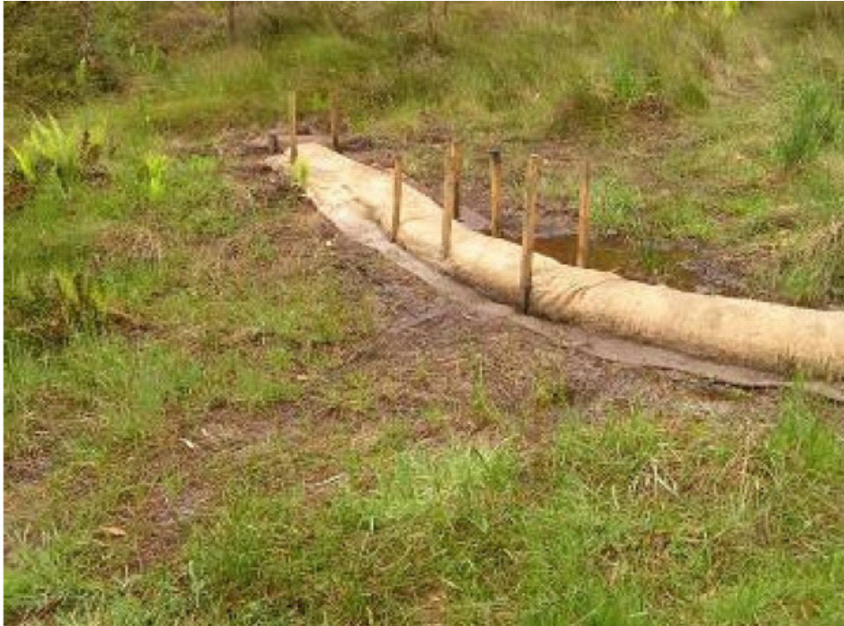
Figure 1 Braeside Swamp condition during installation of coir logs.
