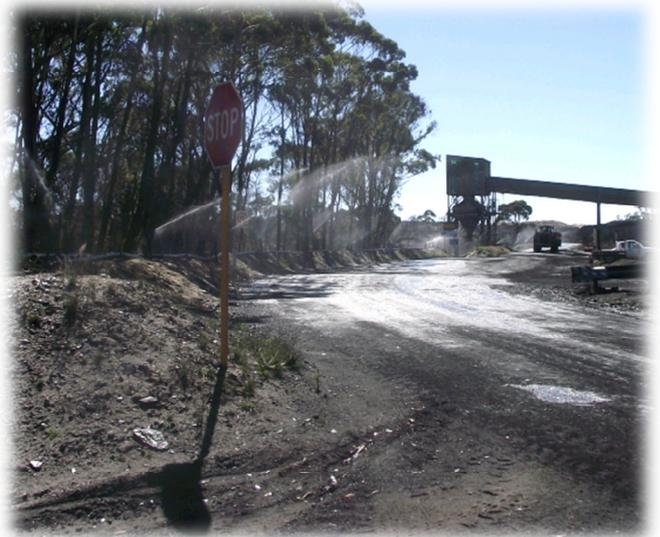
**Figure 7. Upgraded Sprinkler System on Truck Access Road**
