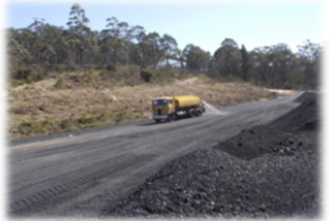
**Figure 6. REA Haul Road Sprinklers and Water Cart in Use at REA IV**
