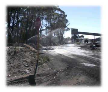
Figure 7. Upgraded Sprinkler System on Truck Access Road
