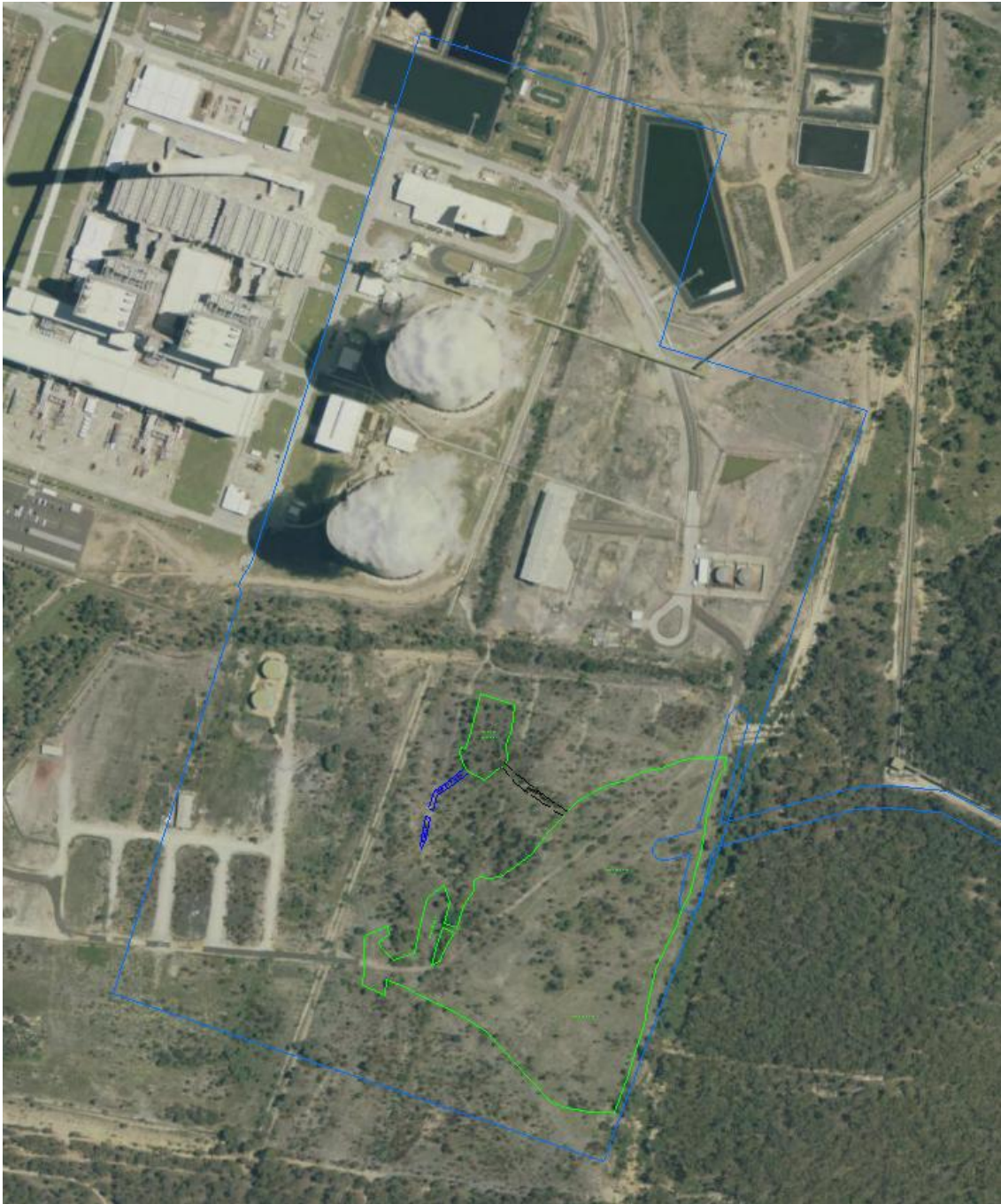
Figure 1.1 : Post-clearing survey of vegetation clearing boundaries undertaken on Friday 15 December 2017 showing area of clearing (green polygons) located within the project application area (Blue polygons)
