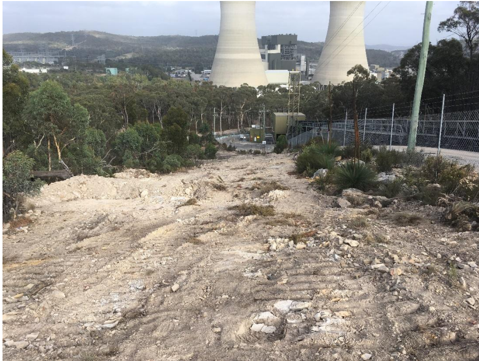
Photo 3 : The project application area at the top of the hill adjacent to the conveyor looking west showing the cleared area and some retained vegetation near the fence
