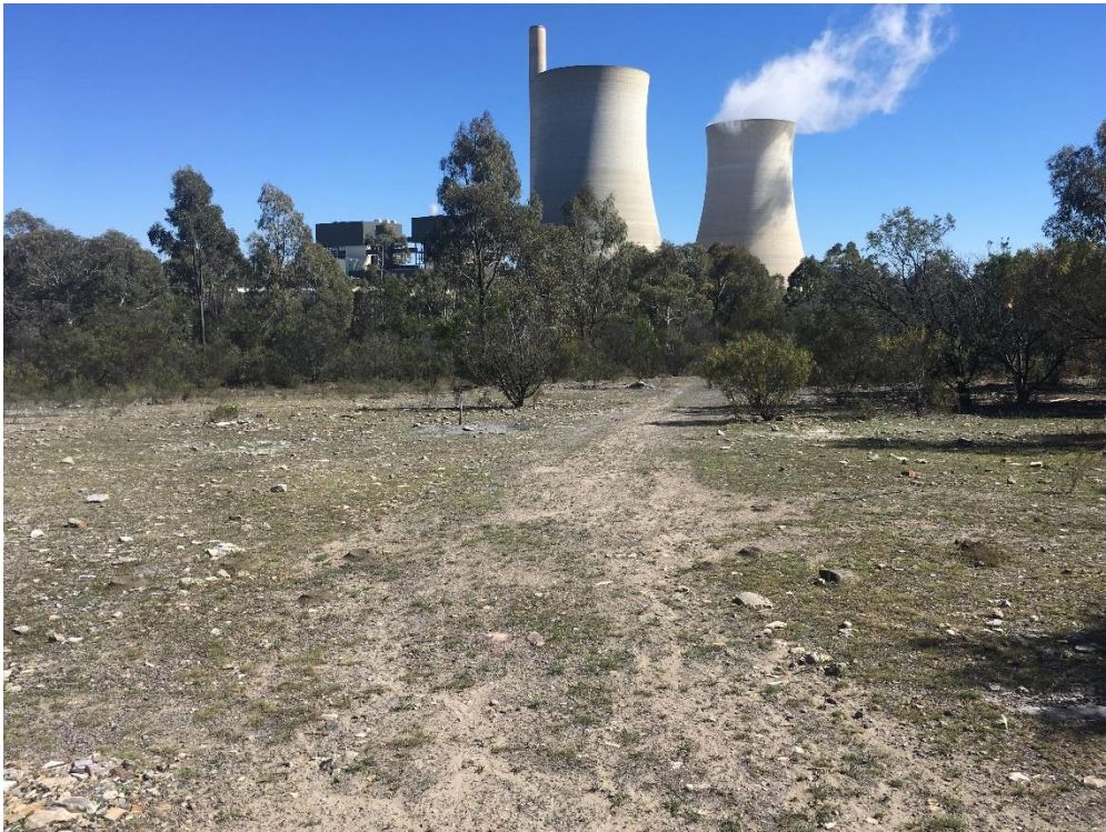
Photo 4: Typical open area within the WTP site with shrub layer in the back ground
