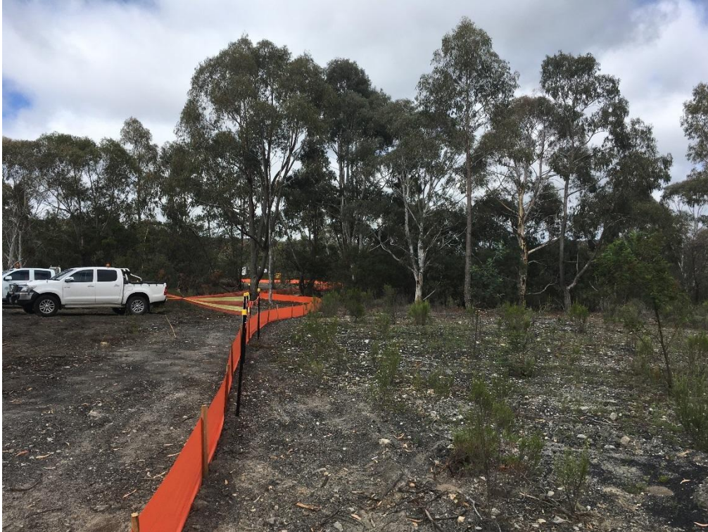
Photo 3: Sediment fencing and exclusion zones have been erected to prevent damage to adjacent vegetation
