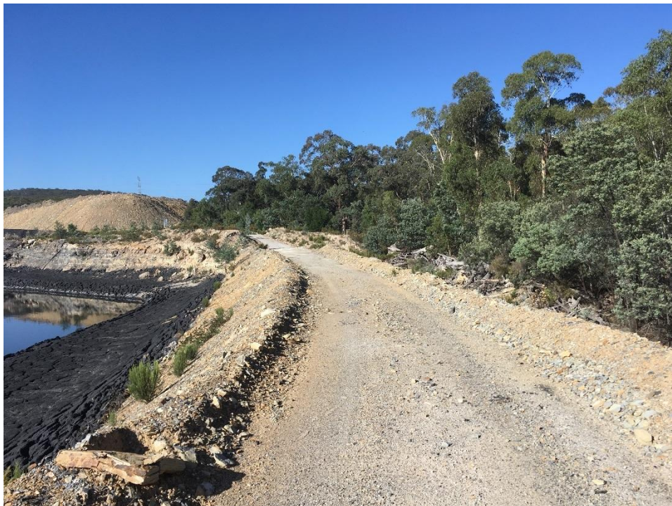
Photo 4 : The project application area along the residuals pipeline showing the road on the outside of the pond where the pipeline will be situated
