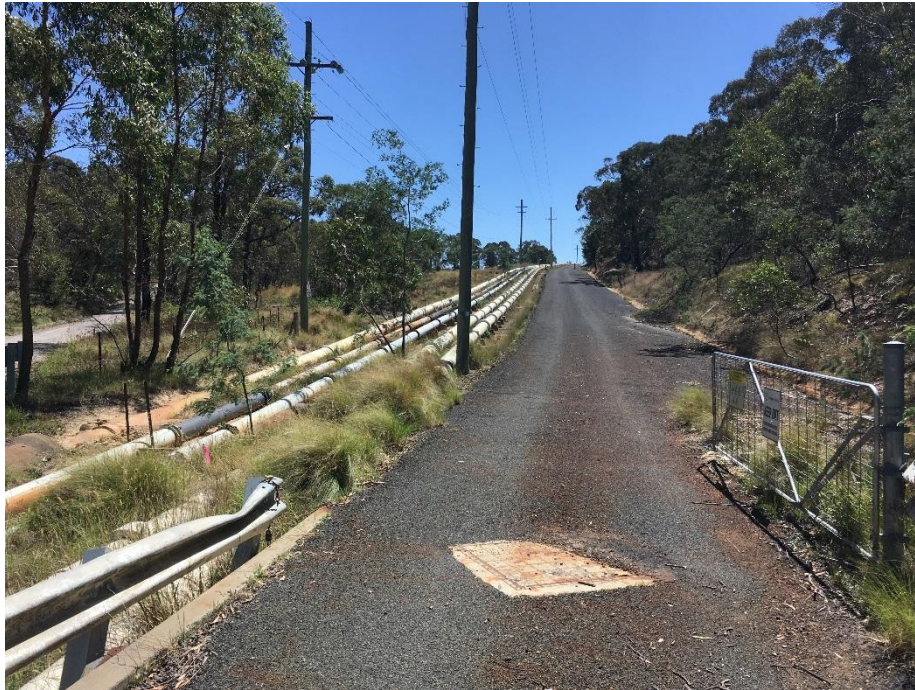
Photo 13 : The disused pipeline and access road in the project application area to the north of Skelly Road
