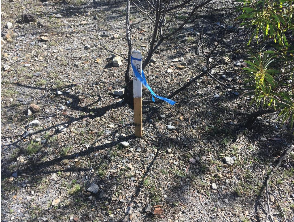
Photo 1: The footprint of the WTP site is marked with survey pegs
