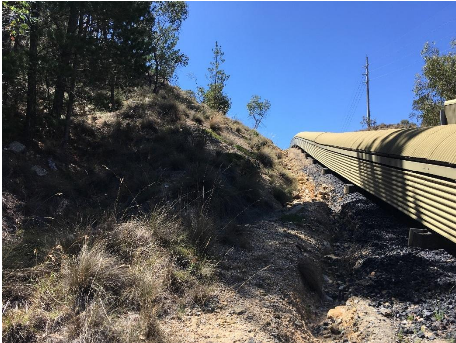
Photo 11 : The conveyor to the east of Wolgan Road in the project application area showing pine forest at the edge of the cutting
