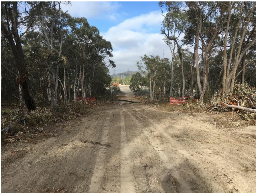
Photo 2 : The project application area east of the WTP site after clearing showing Eucalyptus cannonii trees protected with exclusion zones made from high visibility fencing
