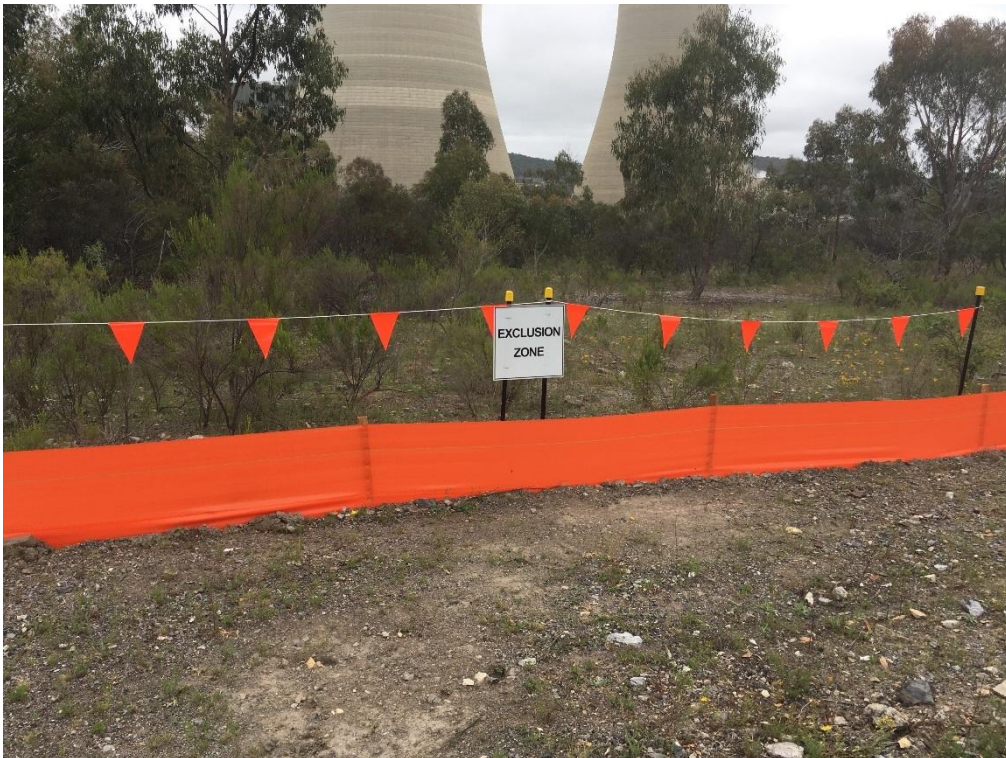
Photo 4: Another example of the exclusion zones and sediment fencing
