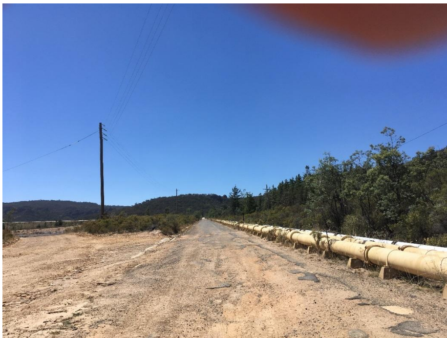
Photo 14 : The old pipeline and access track in the project application area adjacent to the ash dam
