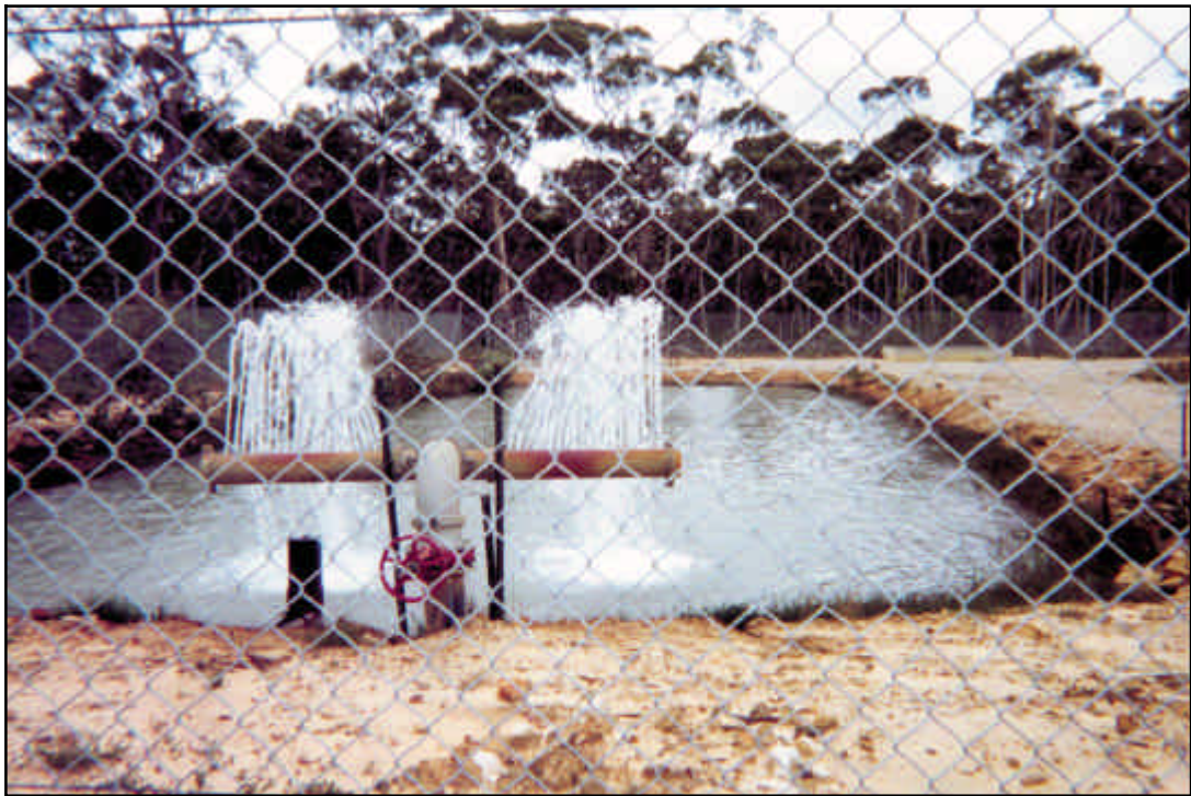
PLATE 3.3 Existing dewatering facility settling pond and aeration facility
