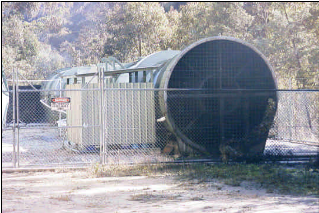
PLATE 3.2 Current Upcast Ventilation Fan Complex
