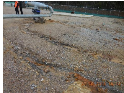
Photo 10. Bore 8 compound. Minor shallow channels in surface
