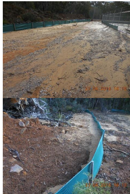
Photo 11. Bore 8 compound. Sediment fence installed parallel to the overland flow and sediment fence with high sediment load downslope of compound
