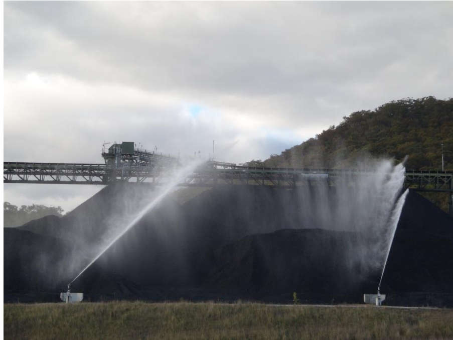
Figure 3 Water Cannons in Operation at Coal Stockpile
