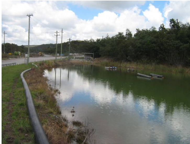
Photo 1: Cooks Dam at Coal Services.
