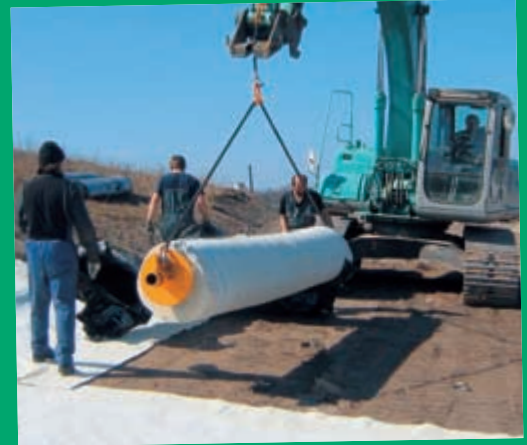
Fig. 2 Bentofix® capping installation
