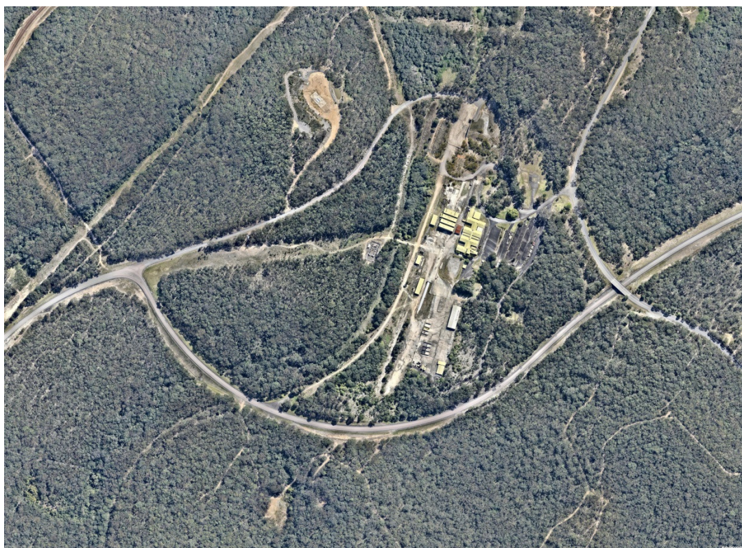
Figure 1: Aerial photograph of Awaba Colliery surface facilities
