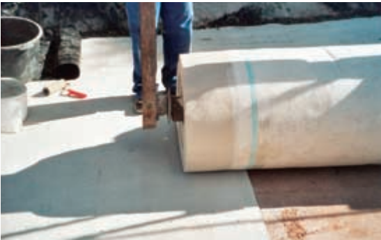
Bentofix® self-sealing overlap
