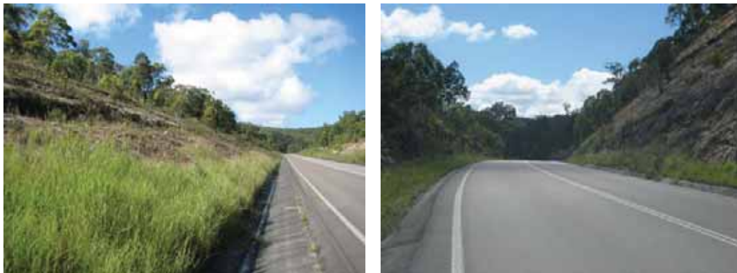
Fig. 6.4 Cutting along the Mine Haul Road (Courtesy of ACOR Appleyard)
