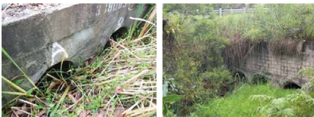
Fig. 6.16 Photographs of Concrete Culverts WA-C1 (LHS) and WA-C2 (RHS) along Wangi Road (Courtesy of ACOR Appleyard)
