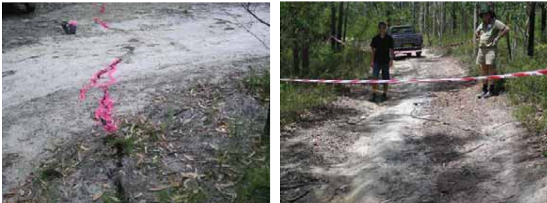
Fig. 4.3 Photographs of Surface Cracking at Newstan Colliery
