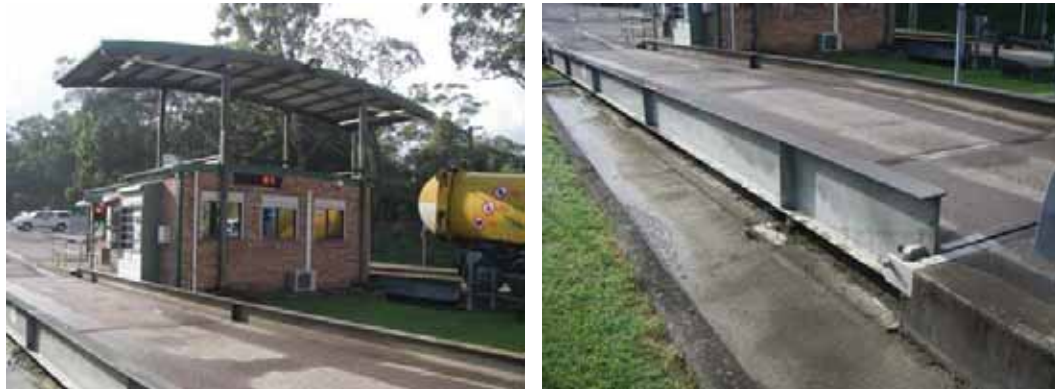
Fig. 6.41 Administration Building and Weigh Bridge (AW002_pa01)
