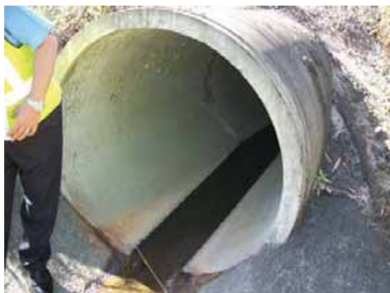
Fig. 6.17 Photograph of Culvert HR-C1 along the Mine Haul Road (Courtesy of ACOR Appleyard)
