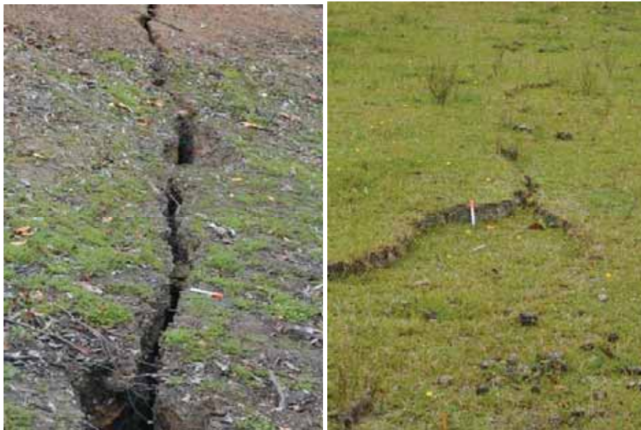
Fig. 4.4 Photographs of Surface Cracking and Stepping at Newstan Colliery
