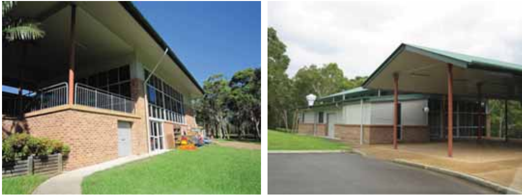
Fig. 6.21 Photographs of the Main Hall (Ref. TR003_pa01) (Courtesy of Northrop Engineers)
