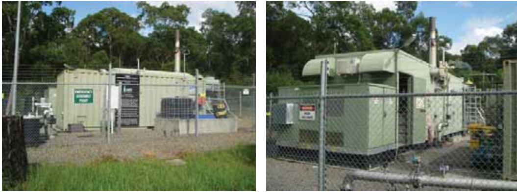
Fig. 6.40 Gas Powered Generation Plant (AW002_pa02 and AW002_pa03)
