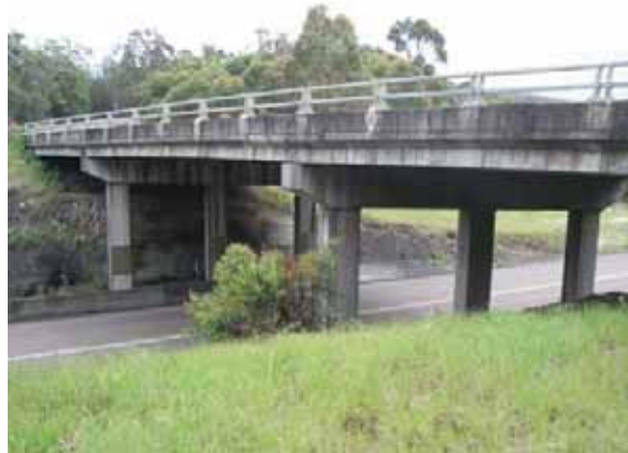
Fig. 6.8 Bridge WR-BR2 where the Wilton Road crosses the Mine Haul Road
