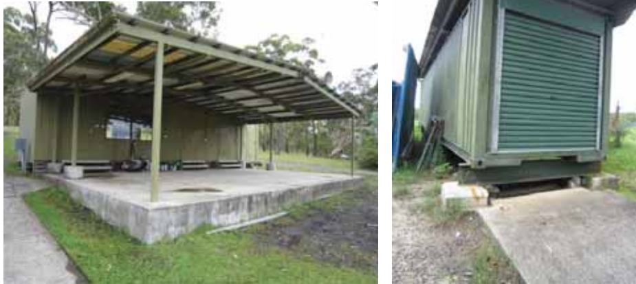
Fig. 6.29 Demountable Structures AW001_pa04 (LHS) and AW001_r15 (RHS) (Courtesy of Northrop Engineers)
