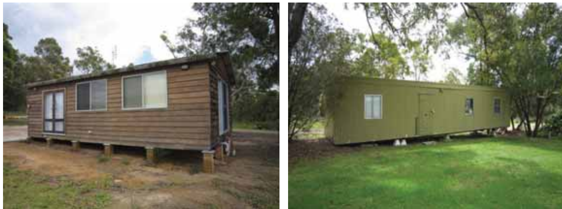
Fig. 6.28 Timber Cottage AW001_pa02 (LHS) and Demountable AW001_pa03 (RHS) (Courtesy of Northrop Engineers)
