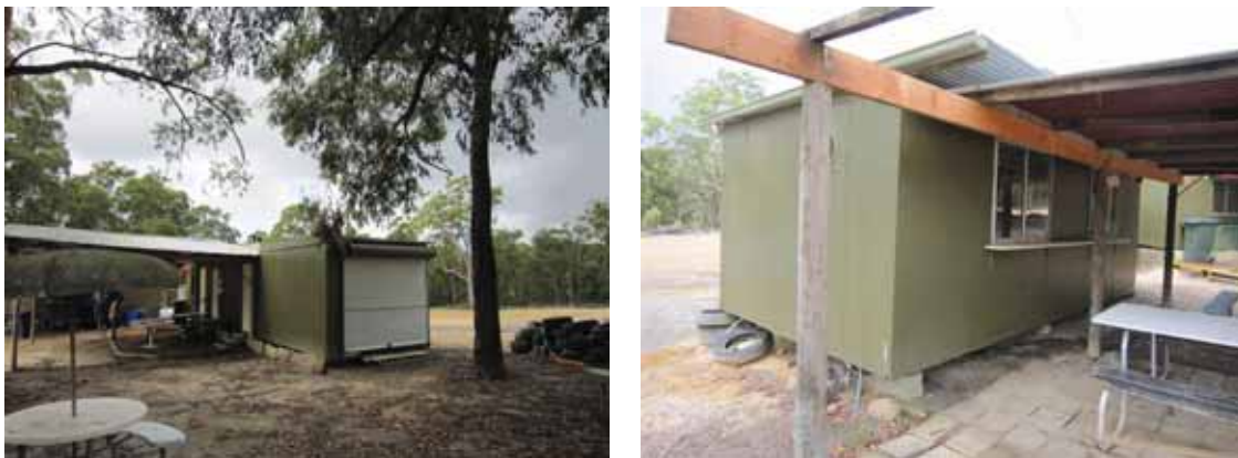
Fig. 6.33 Building Structures at AwabaWAC Park (Courtesy of Northrop Engineers)
