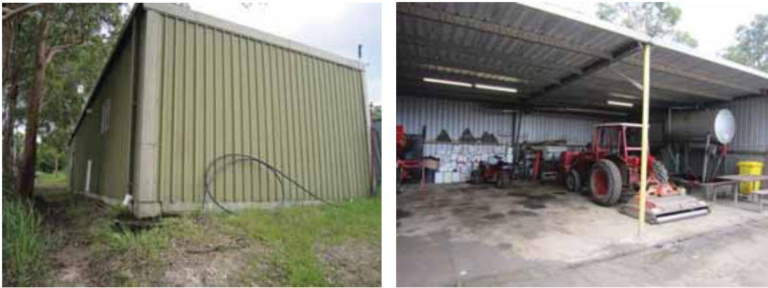
Fig. 6.26 Photographs of the Metal Storage Sheds (Ref. TR001_pa03 to TR001_pa06) (Courtesy of Northrop Engineers)
