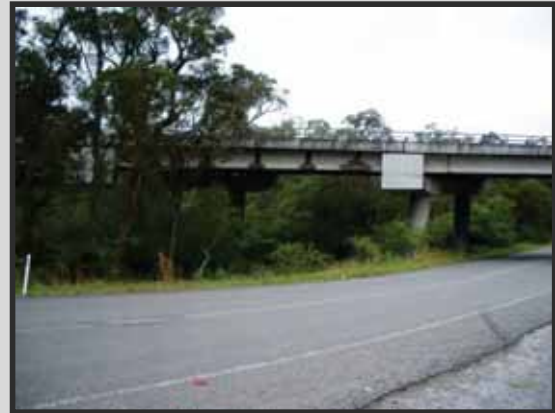
Photo B10 – Stony Creek (WC1) looking upstream from Wilton Road towards Cessnock Road underpass
