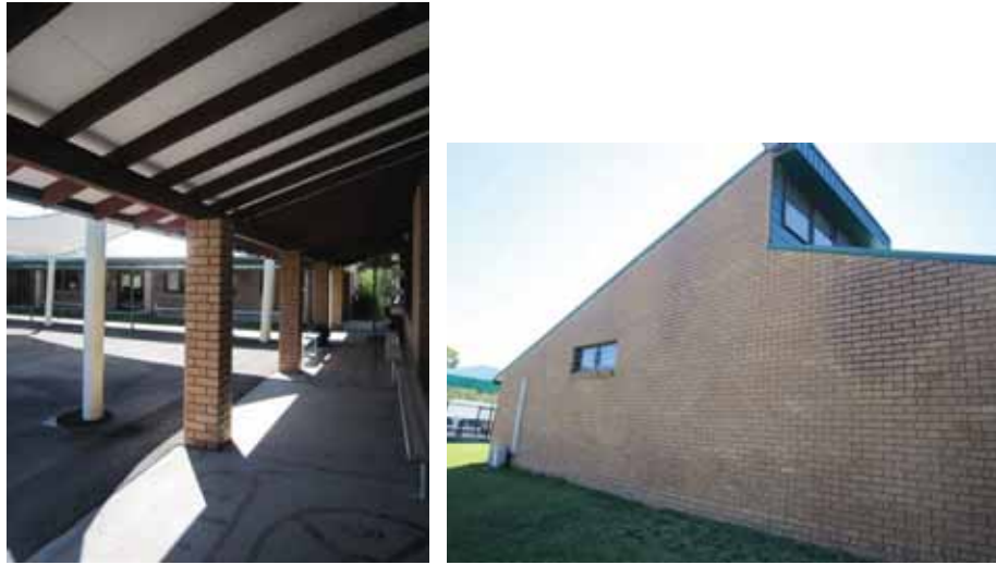
Fig. 6.23 Photographs of Classrooms and Administration Building (Courtesy of Northrop Engineers)
