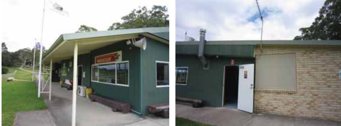
Fig. 6.27 Main Club House (Ref. AW001_pa01) (Courtesy of Northrop Engineers)
