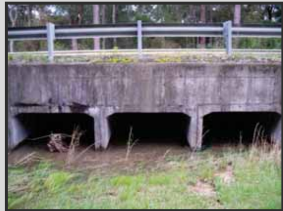
Photo B8 – Kilaben Creek (WC5) culverts under Wilton Road
