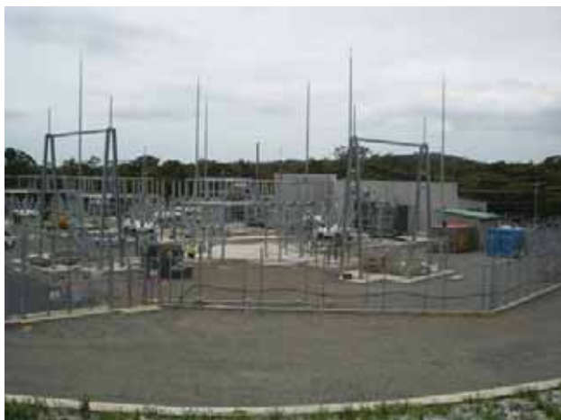
Fig. 6.19 Photograph of the 132/11 kV Substation
