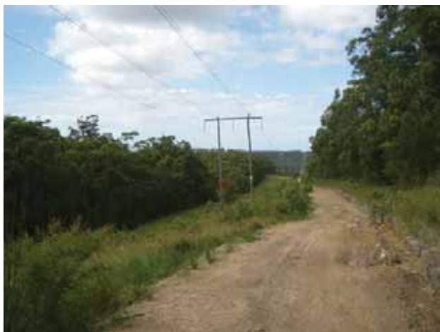
Fig. 6.18 Photograph of a 132 kV Transmission Line
