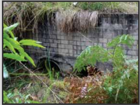
Photo B5 – Kilaben Creek (WC5) Culverts under Wangi Road
