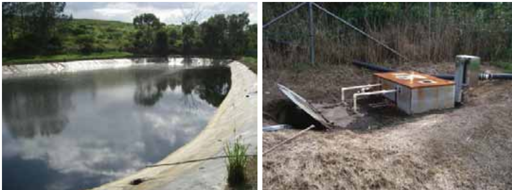
Fig. 6.38 Main Leachate Pond (AW002_d01) and Leachate Well
