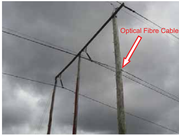
Fig. 6.20 Connection of the AAPT Optical Fibre Cable to a Transmission Pole
