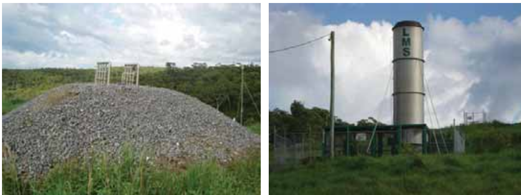
Fig. 6.39 Gas Drainage and Flare
