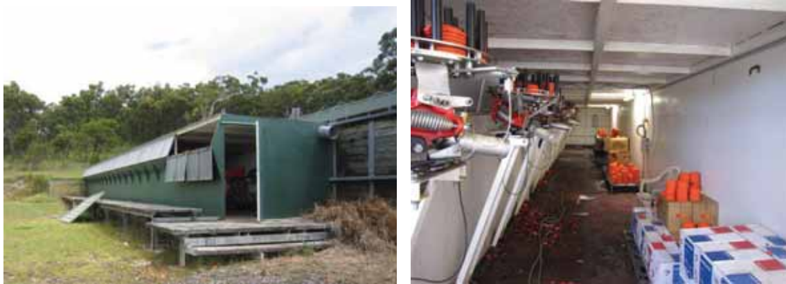
Fig. 6.30 Trap Enclosure AW001_r04 (LHS) and Clay Target Thrower (RHS) (Courtesy of Northrop Engineers)
