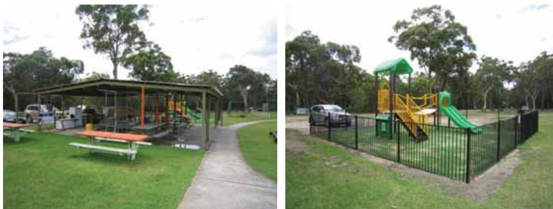
Fig. 6.32 Free Standing Roof Structure (LHS) and Playground (RHS) (Courtesy of Northrop Engineers)
