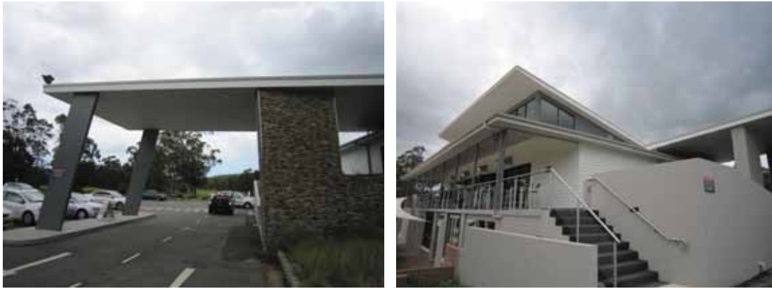
Fig. 6.25 Photographs of the Main Club House (Refs. TR001_pa01 and TR001_pa02) (Courtesy of Northrop Engineers)
