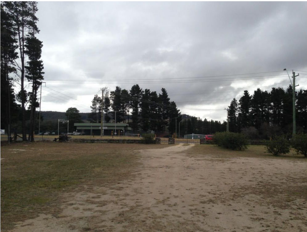
Plate 6: Lidsdale Siding facility viewed from St John's, looking north.
