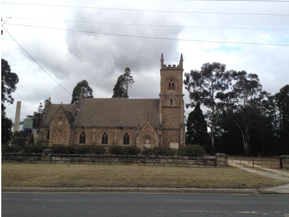
Plate 1: St John the Evangelist, Wallerawang, looking south. Part of Wallerawang Power Station can be seen at far left.
