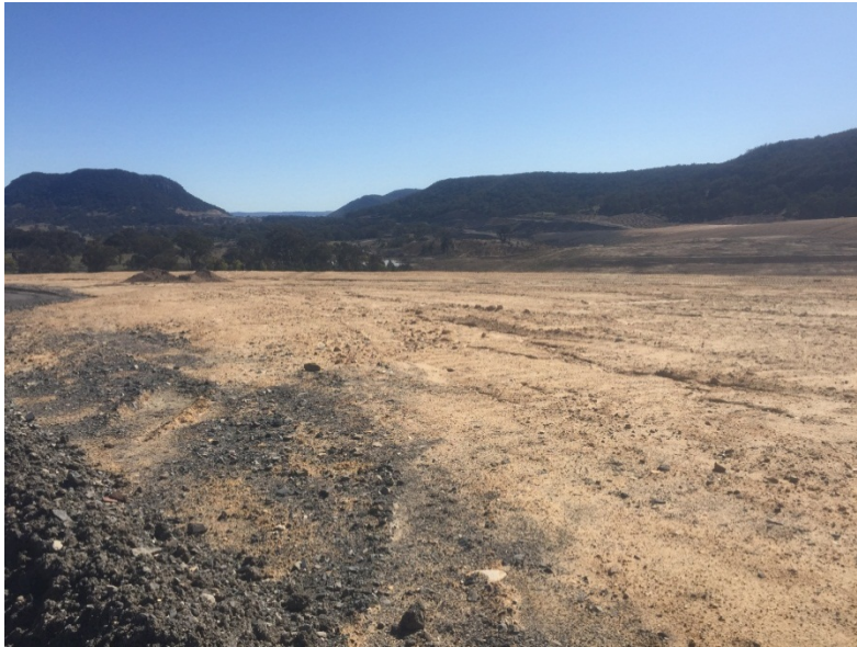
Example of final landform shaping undertaken prior to planting
