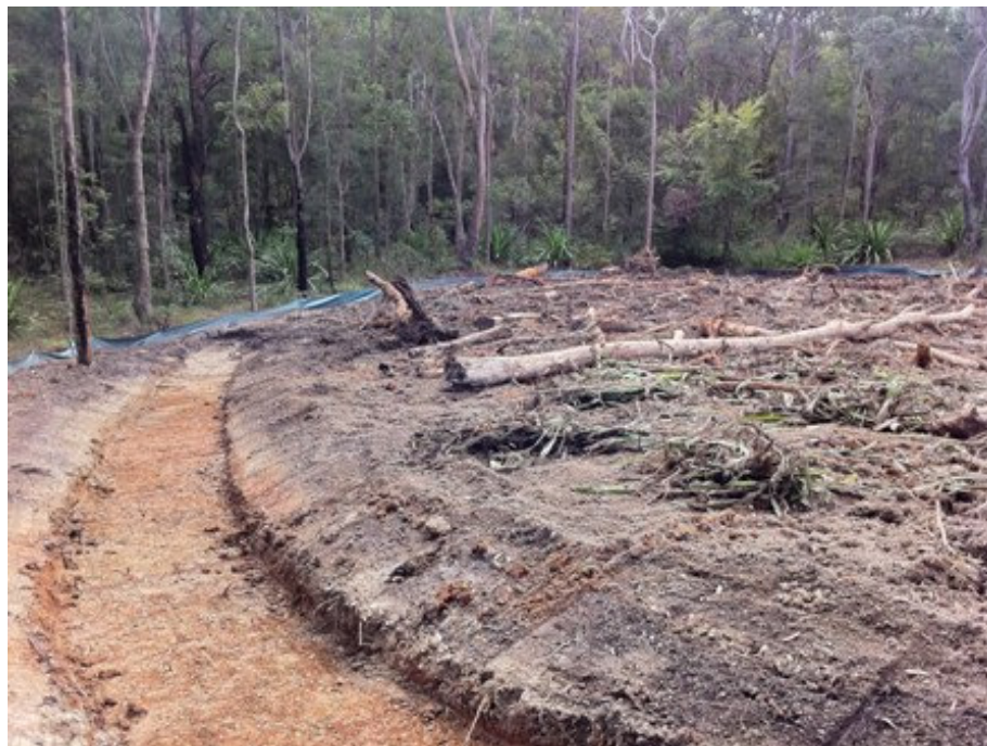
Figure 9: Replaced top soil and vegetation and surrounding water diversion drains.
