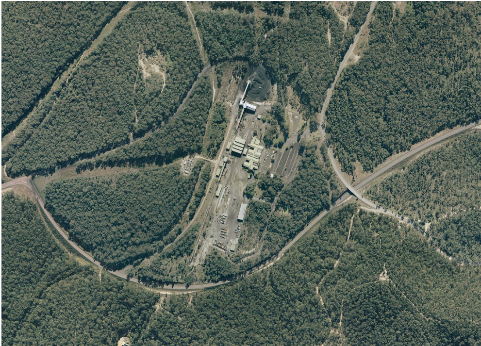
Figure 1: Aerial photograph of Awaba Colliery Surface Facilities
